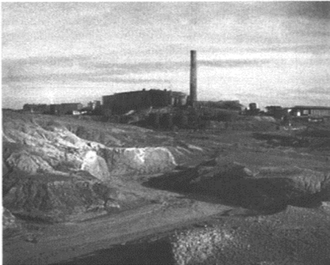
Fig. 7.3 “A Model example of the transformative techno-fix, the Ducktown sulfuric acid plant removed a large part of the sulfur dioxide fumes produced in smelting copper and transformed it into a new product that was valuable for manufacturing fertilizers and many other industrial processes.” (Library of Congress, Prints & Photography Division, FSA-OWI Collection, Reproduction Number LC-USF34-052180-E DLC.)
