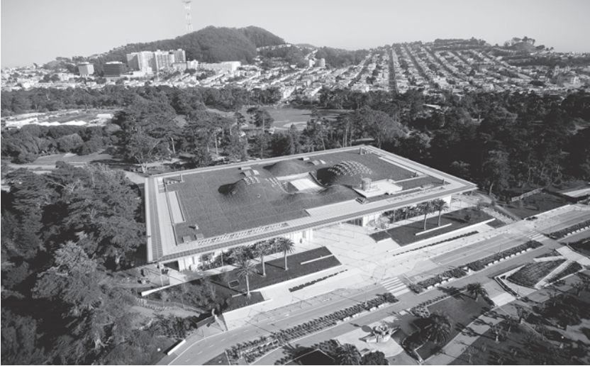
FIGURE 10.3 The 1-hectare (2.5-acre) green roof of the California Academy of Sciences in San Francisco is part of the green spaces in the densely populated city. (© 2008 California Academy of Sciences.)
