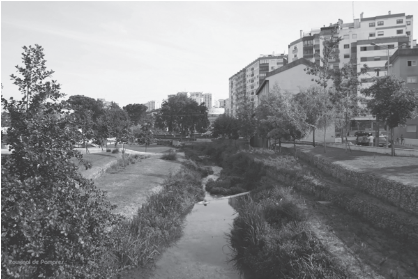
FIGURE 10.5 The condition of the Ribeira das Jardas near Lisbon, Portugal, before (above) and after (below) the rehabilitation project. (Photos by Graça Saraiva and António Manuel Silva.)
