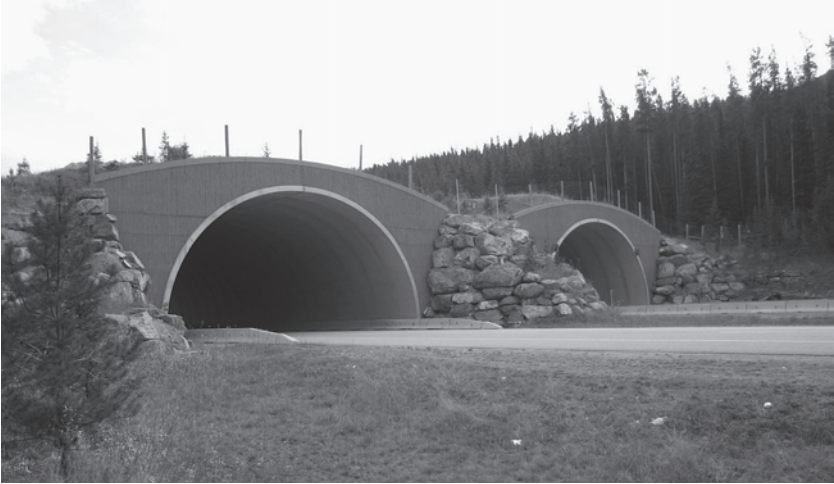
FIGURE 5.3 Wildlife overpass across the Trans-Canada Highway, one of six established to increase connectivity for populations of wildlife in Banff National Park, Alberta. (Photo by Jodi Hilty.)
