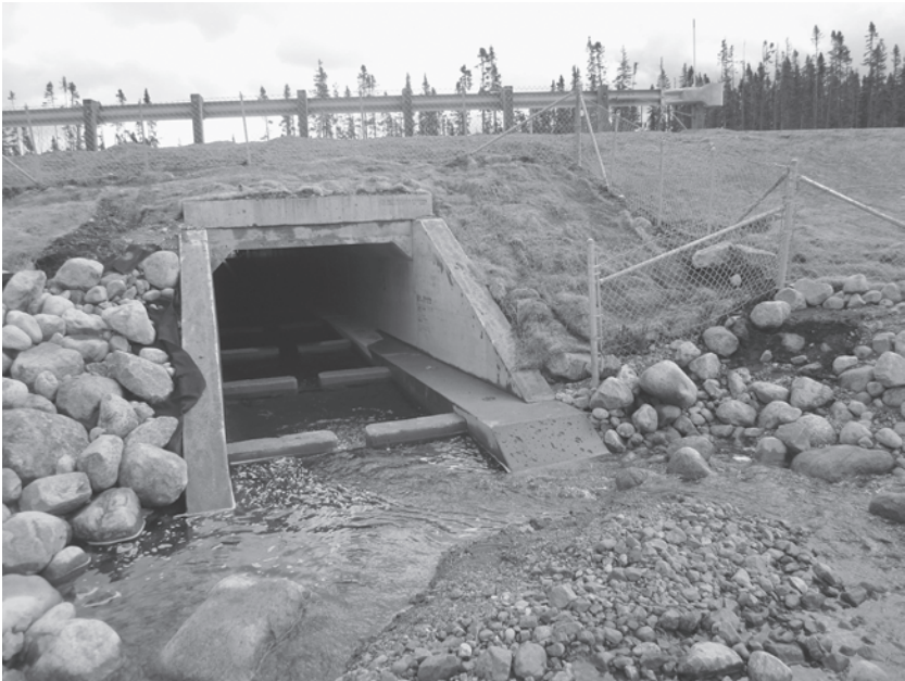
FIGURE 7.6 Culverts with ledges or walkways will retain functionality for connectivity even if flooded. (From Jaeger et al. 2017.)
