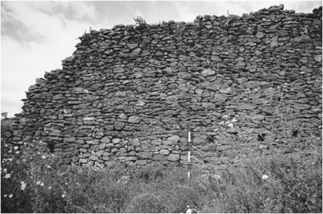
4.2. Standing wall fragment showing both horizontal and vertical seam.
