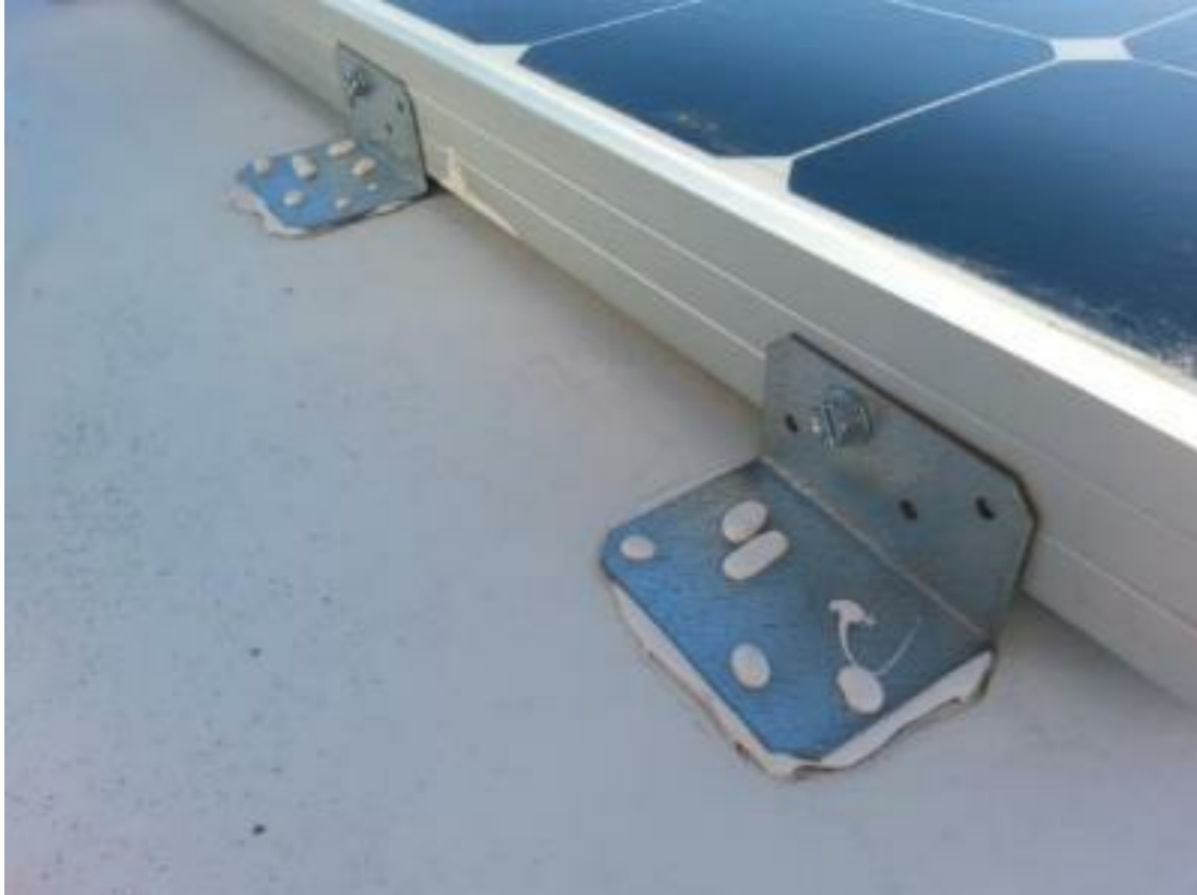
Mounting solar panels on RV roof with brackets Source: JdFinley.com
