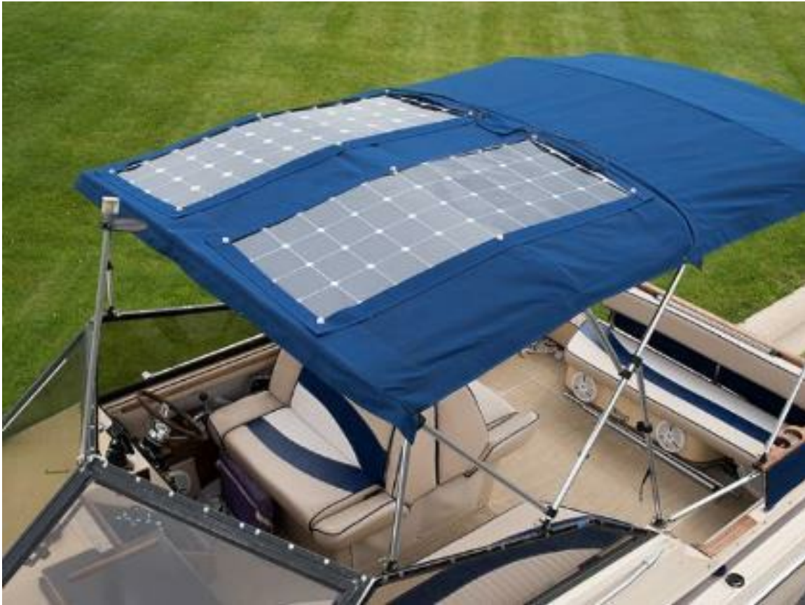
Installing solar panels on a Bimini
