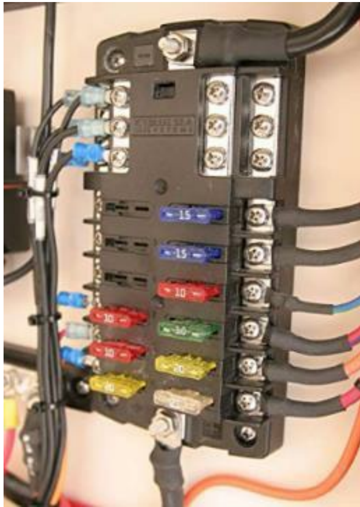
Wiring of a DC fuse box using spade fuses Source: Blue Sea Systems
