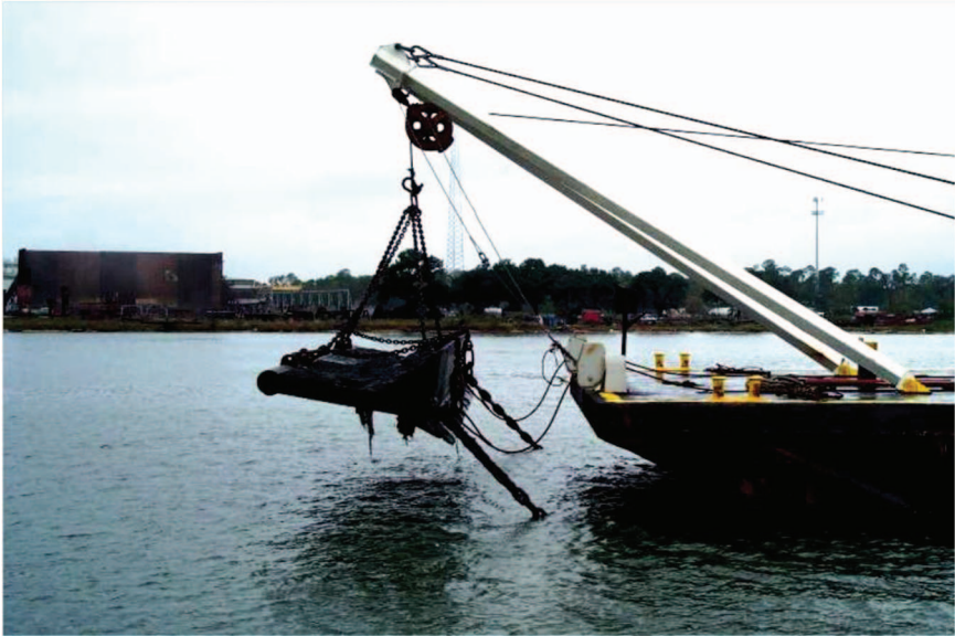
Figure 9-4. Bed leveler suspended by an A-frame on a work barge.
