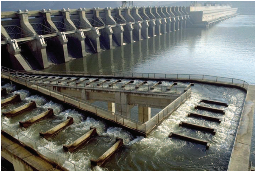
Figure 11-5. John Day fish ladder. Source: USACE, Portland District.
