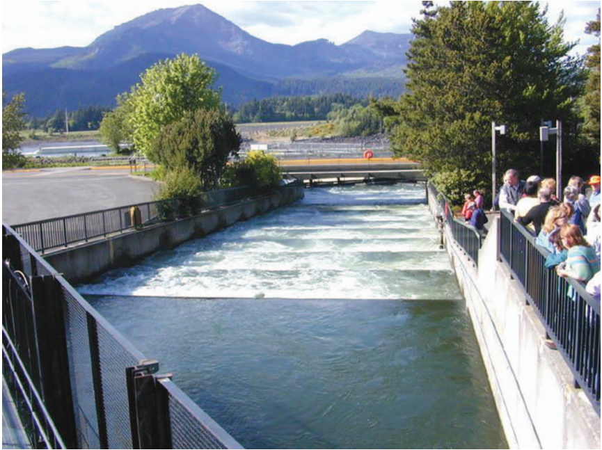
Figure 11-4. Bonneville Dam fish ladder. Source: USACE, Portland District.
