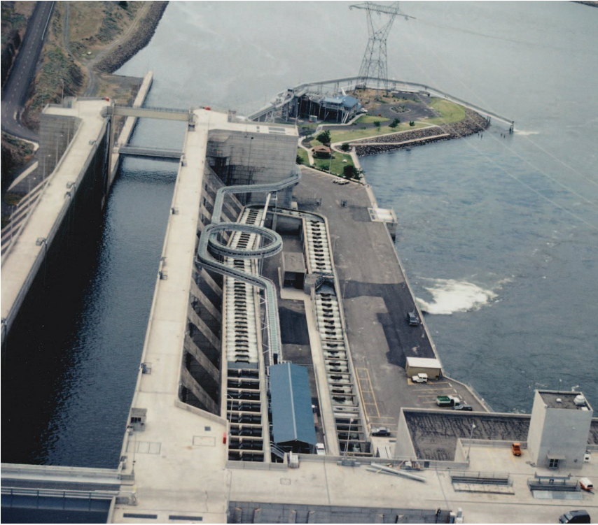
Figure 11-7. Little Goose Dam fish bypass.
