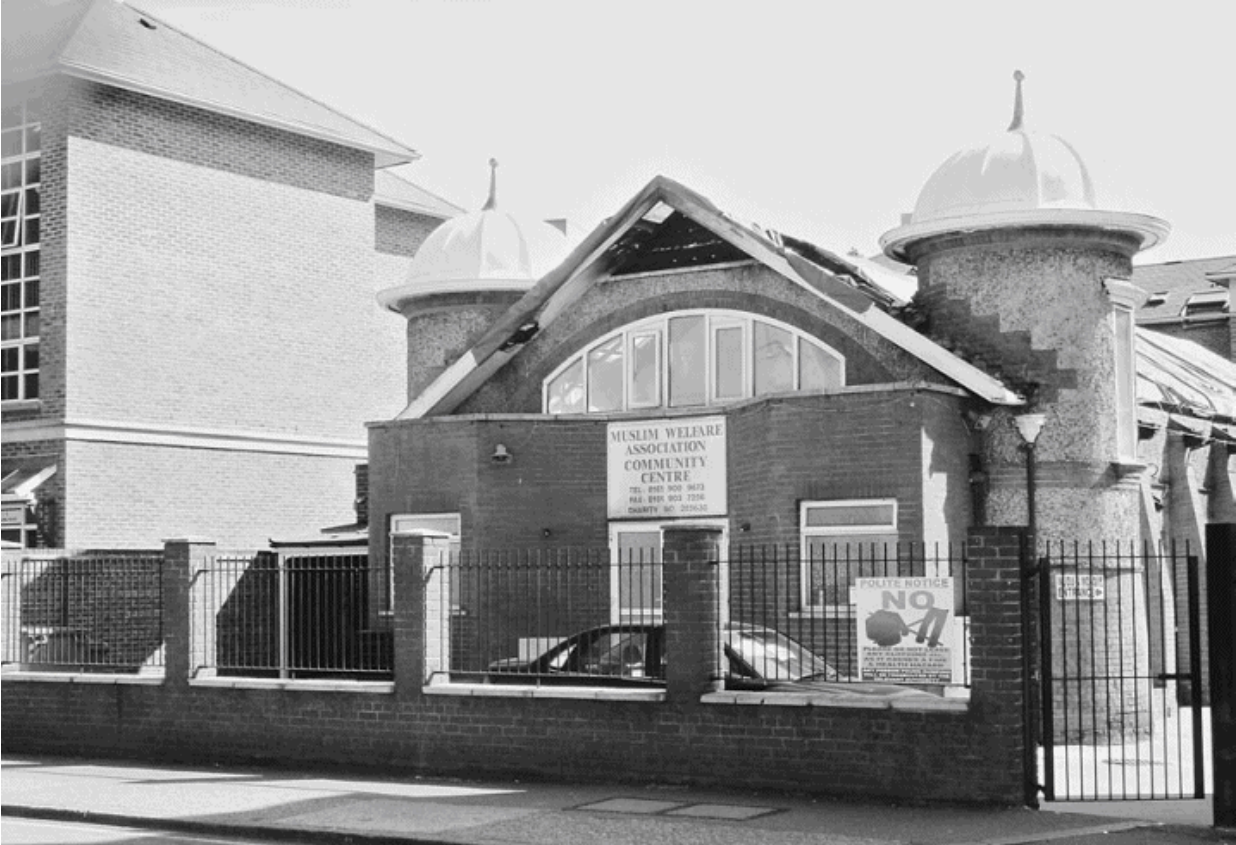
Suburban London mosque, formerly a church ( J. Gordon Melton )
