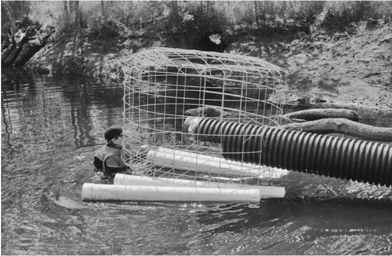
Figure 13.1. Pond leveler installation to mitigate flooding by beavers. G. A. HOOD
