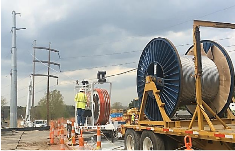
Figure 3-2. Wire stringing operations and vertical and transverse load at snub structure.
