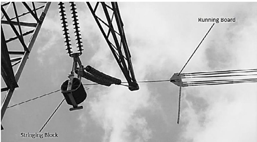
Figure 3-5. Wire stringing operations.
