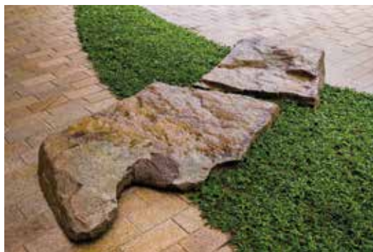
TOP At the intersection of several paths faced in rectangular and square stone pavers, odd-shaped stones fit tightly together like an overscaled mosaic.
