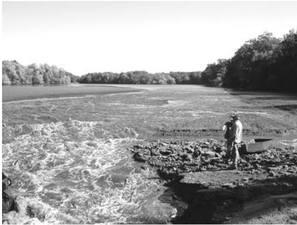
FIGURE 11.21 Dam removal on Koshkonong Creek, Rockdale Wisconsin in 2000. The remnants of a low dam are visible in the foreground. The stream is cutting through and resuspending the fine mud sediments that had accumulated behind the dam. Source: photo Dscn0143 by Martin Doyle.
