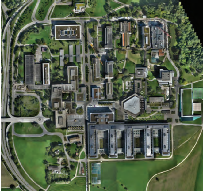
Figure 5.11 Orthoimage from the Campus Science City ETH Zurich, generated from R-Pod UAV images during the UAV-g conference in 2011 ( www.uav-g.ethz.ch/ ).
