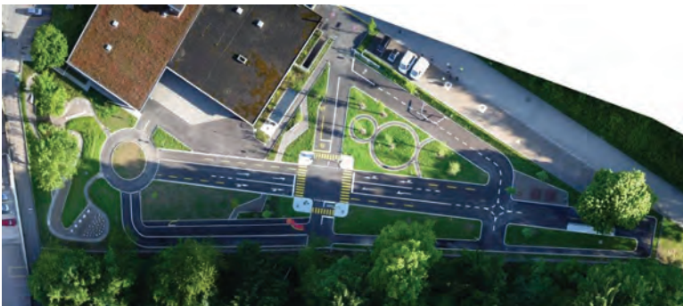
Figure 5.2 Traffic education area of city of Winterthur (2012, 3 cm ground sampling distance (GSD)).
