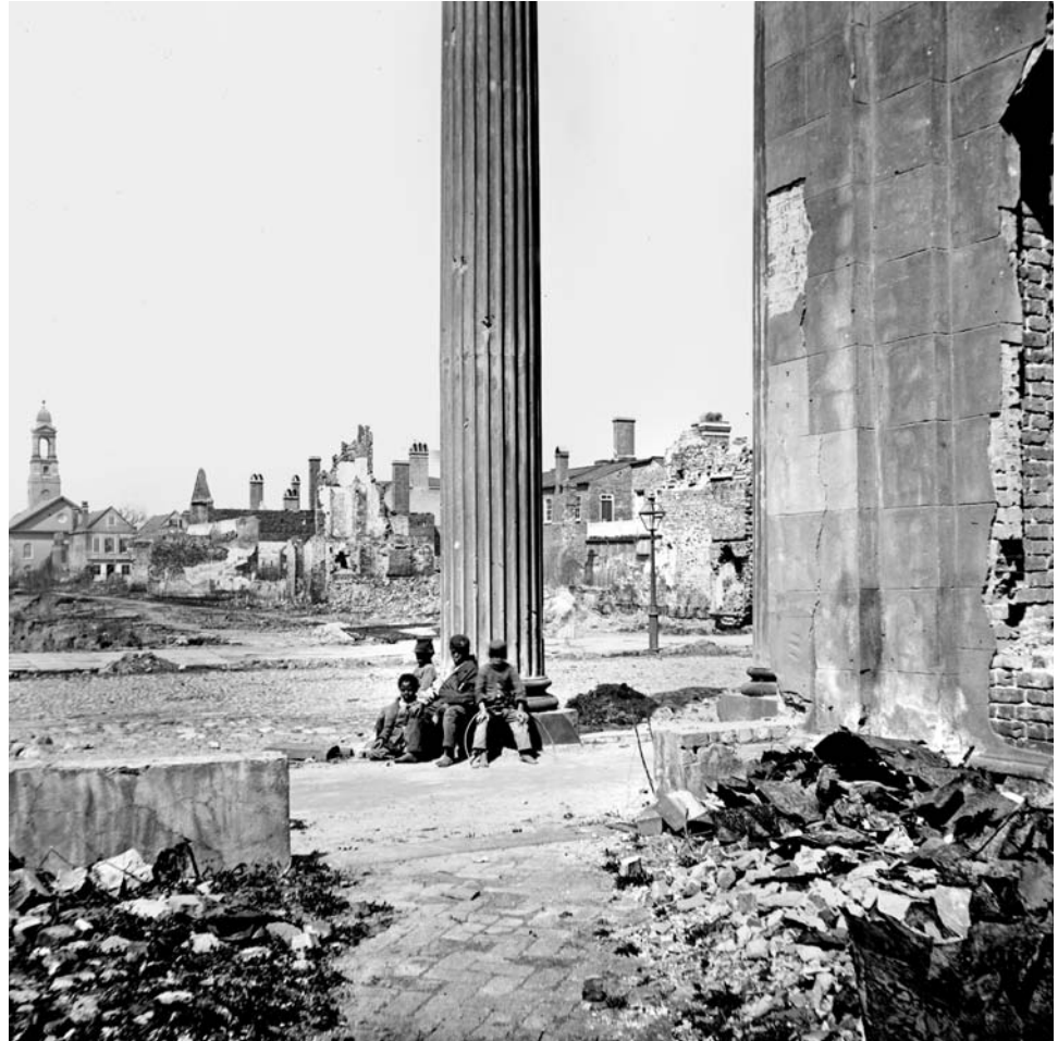
At the end of the war, many of Charleston's buildings were damaged or destroyed from Union artillery fire. Children played among the ruins of the Circular Church, 150 Meeting Street. ( Library of Congress, Prints and Photographs Division, LC-B8171-3448 )
