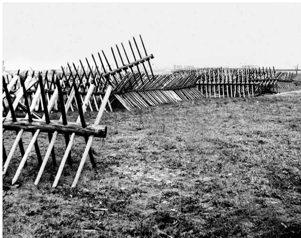
Sharpened wooden stakes, or chevaux-de-frise were employed by both sides as defensive fortifications in the field. ( Library of Congress, Prints and Photographs Division, LC-DIG-cupb-02602 )
