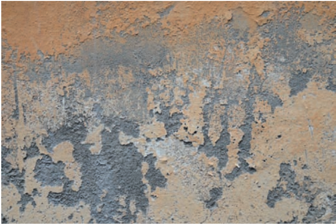
FIG. 2-25 Italian stucco wall.
