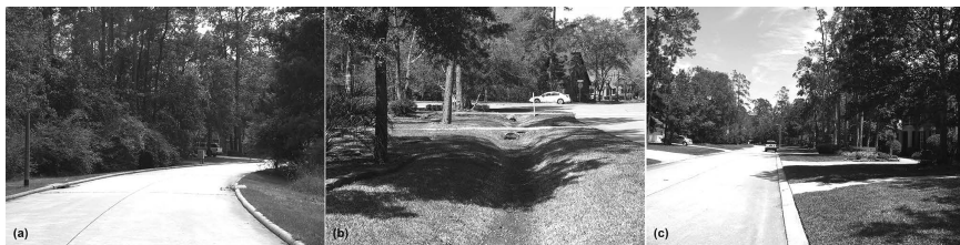
Figure 16.2 Different drainage solutions and landscaping types in The Woodlands, before and after 1997 ownership change.
