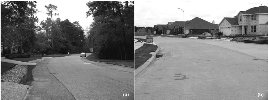
Figure 8.2 Typical neighborhood views in (a) The Woodlands (McHarg’s ecological design: curbsless streets, open surface drainage, and well-preserved vegetation) and (b) comparative Houston communities (curb-and-gutter conventional drainage and less consideration of preserving vegetation).
