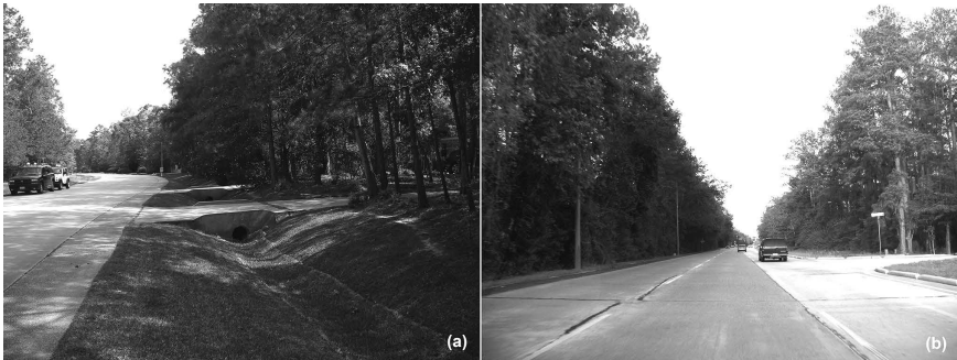
Figure 6.1a A neighborhood street view in Grogan's Mill, the first subdivision village of The Woodlands. Unlike conventional development, McHarg used narrow and curbless streets, with open surface drainage, mandated to preserve the original vegetation after development.
