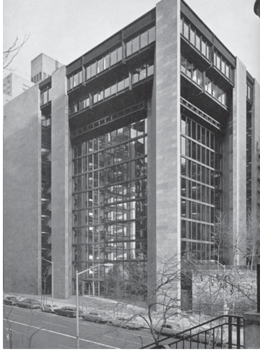
4.14 Classic, fully- conditioned, atrium building with return air circulated through atrium space and plantings. Ford Foundation, 1968. 43
