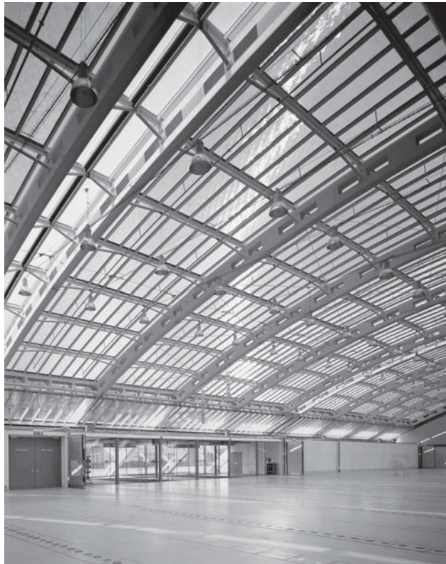
5.12 Design Center: steel girders framing the roof structure.
