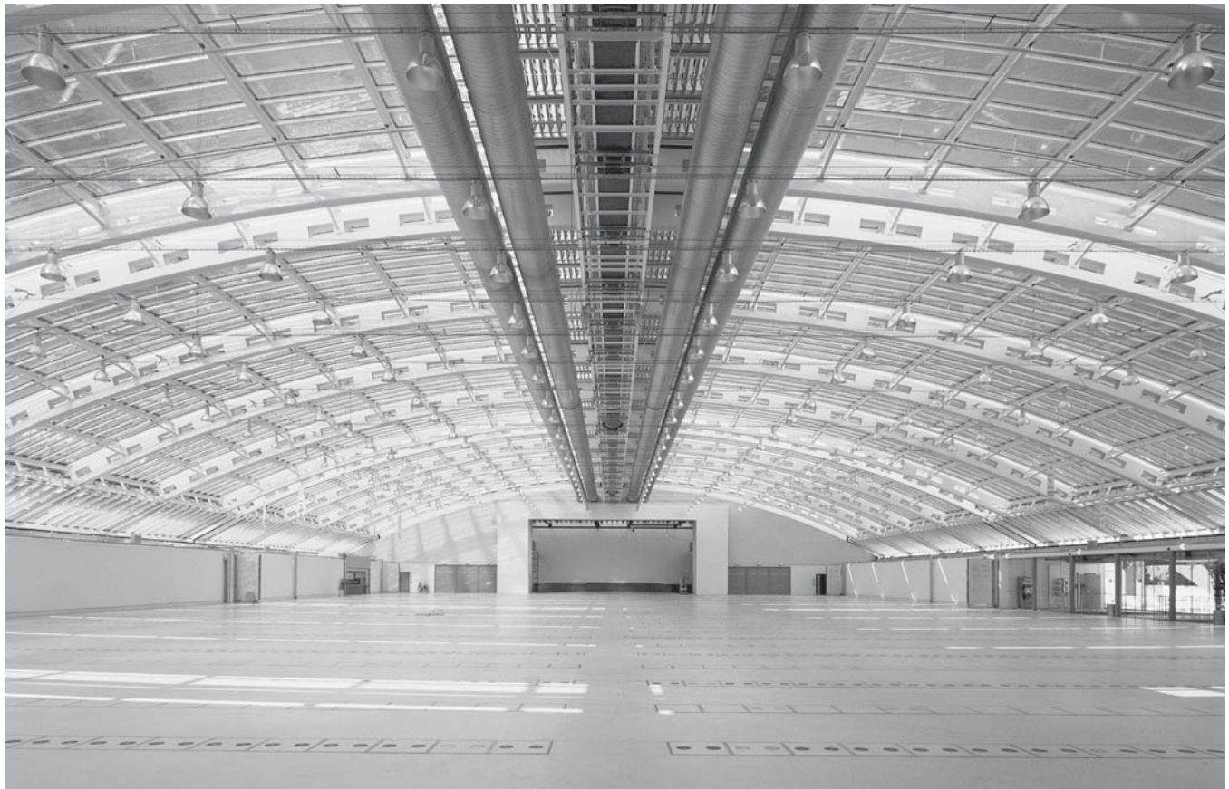
5.10 Design Center: exhibition hall with the ventilation system.
