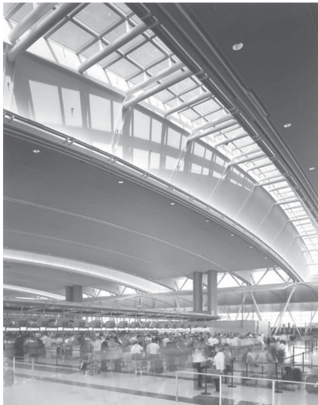
3.12 JFK Terminal 4: linear skylights provide daylighting.
