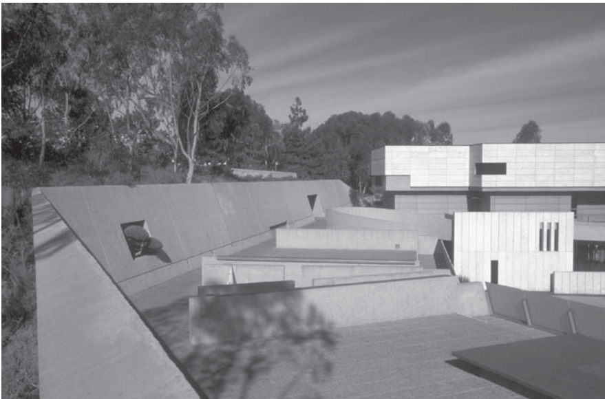
1.8 The upper deck, Neurosciences Institute, La Jolla, California (1992–95), architects Tod Williams and Billie Tsien.
