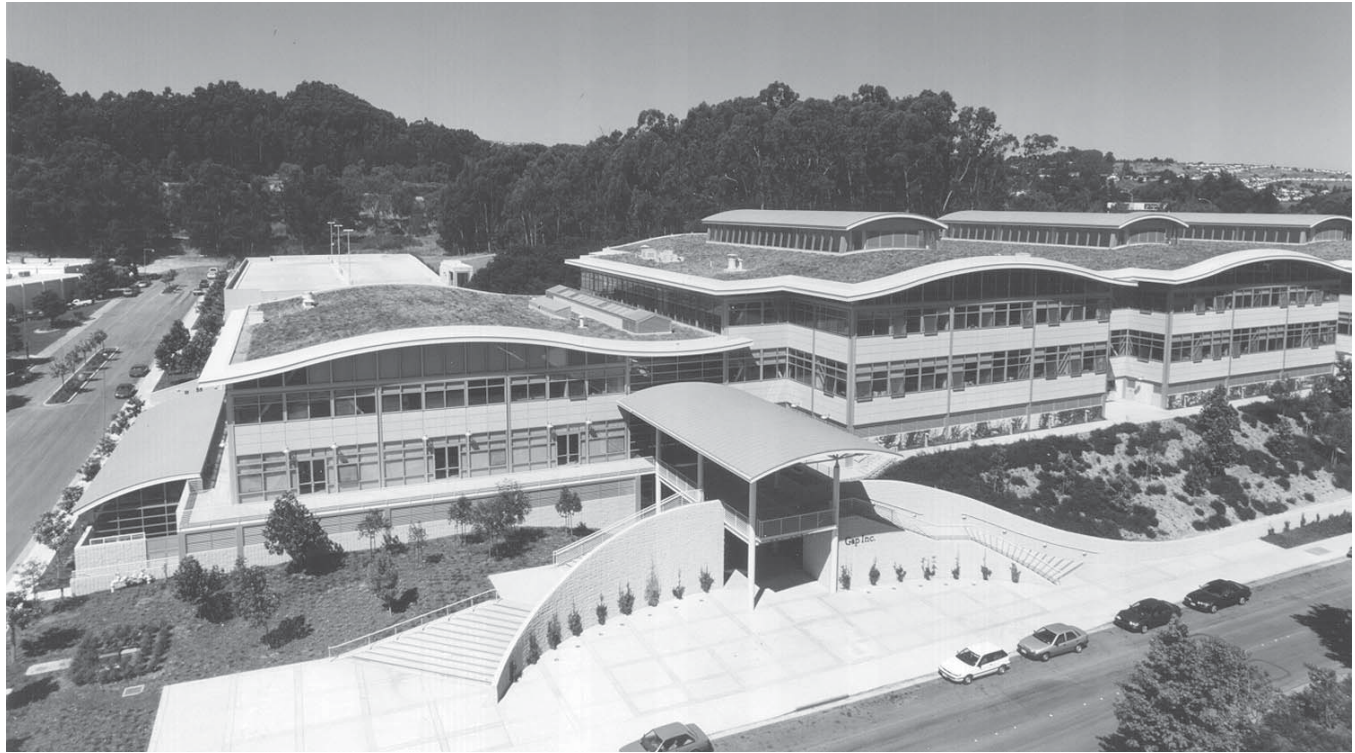
3.3 GAP Headquarters, San Bruno, California (1996–1998), architects William McDonough + Partners and Gensler.
