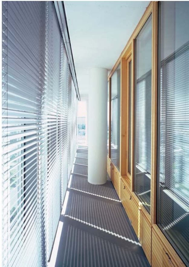
5.34 DMAG: intermediate space between façade skins.
