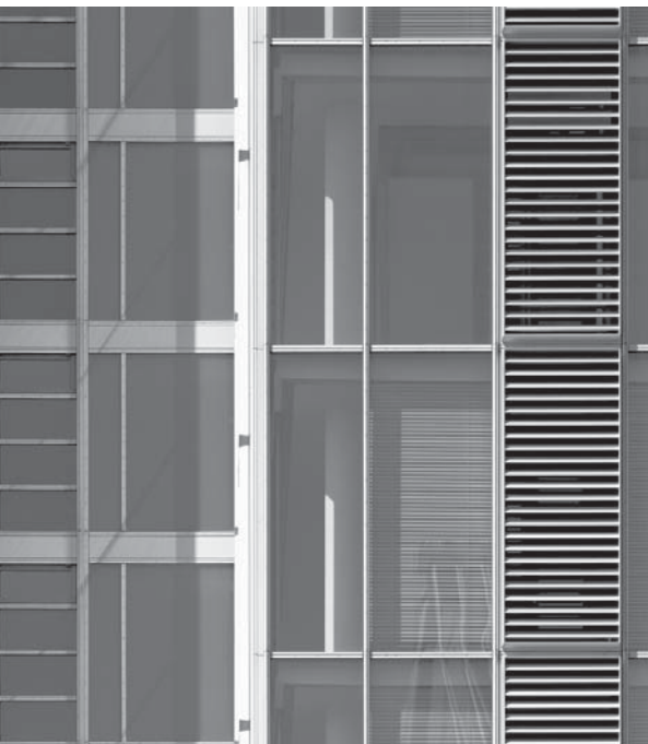
5.31 DMAG: double-skin façade with fixed glazing.
