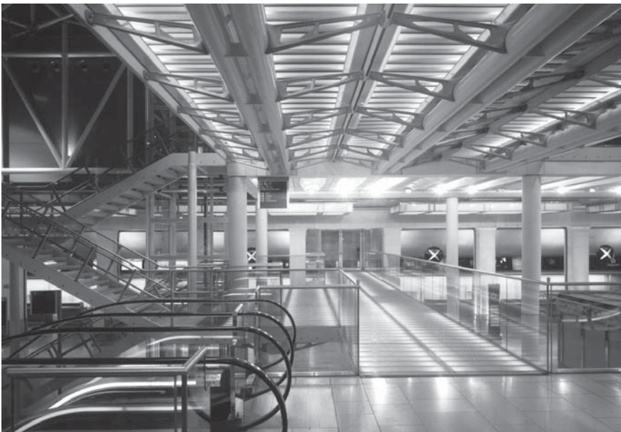
2.11a–b Paddington Station, London (1997–99), architect Grimshaw.
