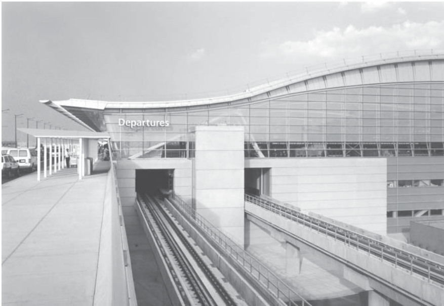
3.12 JFK Terminal 4: linear skylights provide daylighting.
