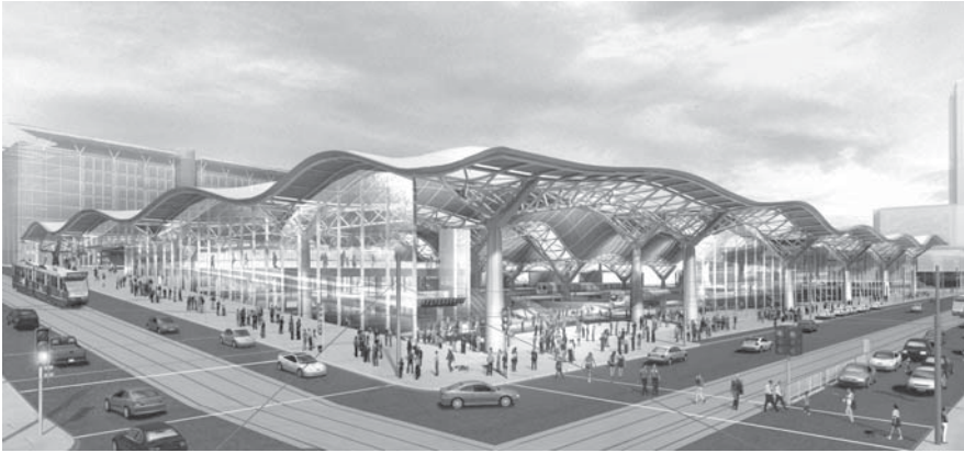
2.28 Southern Cross Railway Station, Melbourne, Australia (2002–), architect Grimshaw.
