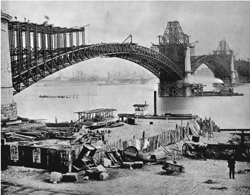
Eads' Bridge under construction. Library of Congress.
