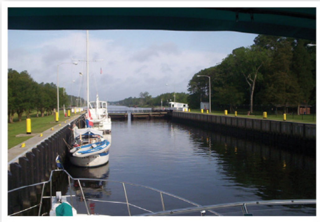
Great Bridge Lock – Atlantic Intracoastal Waterway
