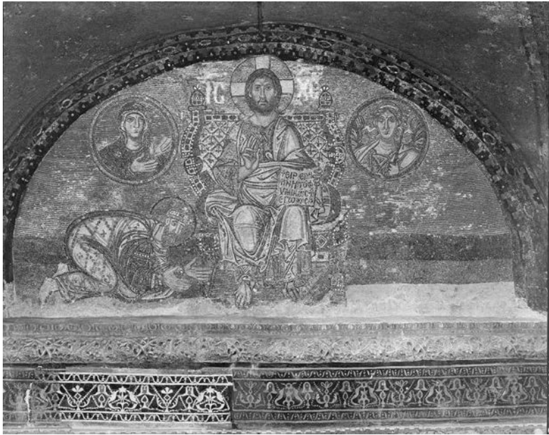
Fig. 17.4 Narthex mosaic of emperor before Christ, Istanbul, Hagia Sophia, c.900. Photography courtesy of Dumbarton Oaks, Washington, DC
