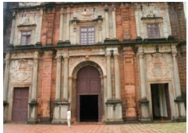
Fig. 5. 106. Old Goa. Basilica of Bom Joseph. Lower divisions of façade. 1594-1605. Laterite and mortar.
