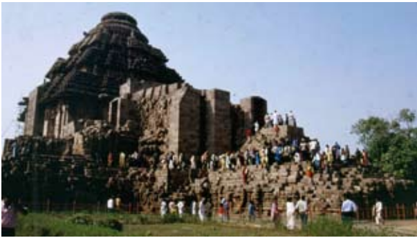
Fig. 4.67. Konarak. Sun Temple. Collapsed deul. 1238-1264. Laterite, Khondalite, Chlorite.
