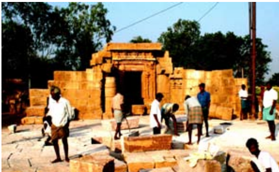
Fig. 2.123. Patadkal. Jain Temple. Dismantled porch. Sanctum in the rear. Ca. 9 th Century. Sandstone
