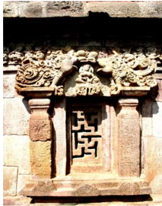
Fig. 2.88. Kadlur. Sangameshvara temple. Temple wall. Window. Ca. 6 th Century. Sandstone.
