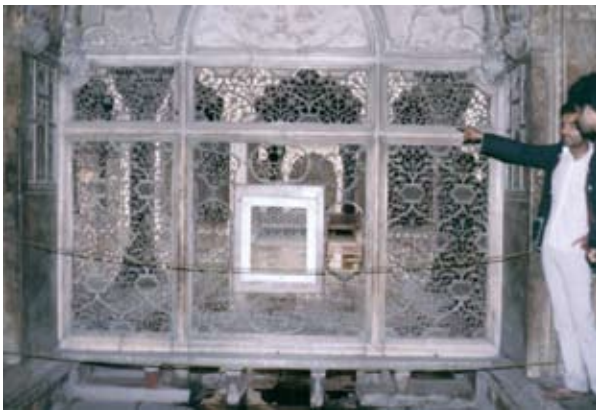
Fig. 5.19. Delhi. Red Fort. Khas Mahal. Marble screen above the stream. 1639-1649. Marble.
