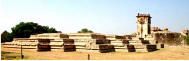
Fig. 4.104. Vijayanagara. Zanana enclosure. Foundation of Queen's palace. Ca. 1334-1565. Granite.
