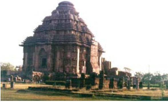
Fig. 4.52. Konarak. Sun Temple. Jagamohan and collapsed rekha deul. 1238-1264. Laterite, Khondalite, Chlorite.
