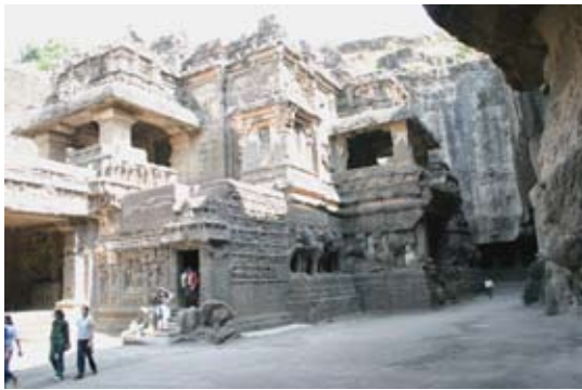
Fig. 2.161. Ellora. Kailas Cave 16. Mandapa connected to Bull pavilion in front. Ca. 750-800. Basalt.
