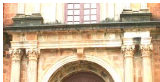
Fig. 5.103. Old Goa. Churches. Pilaster orders. (A) Corinthian, (B) Doric, (C) Ionic (D) Composite - Basilica of Bom Joseph. (E) Tuscan - Church of St. Francis of Assisi
