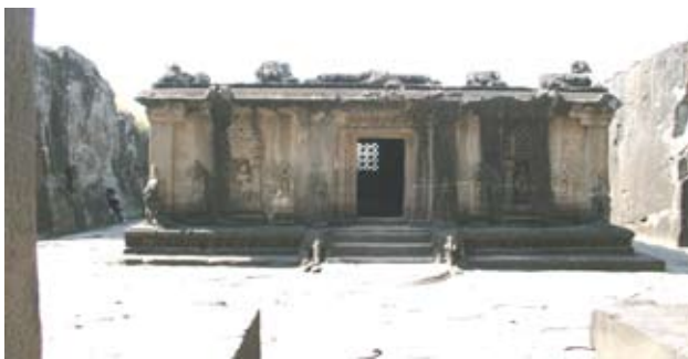
Fig. 2.155. Ellora. Cave 15. Monolithic hall in verandah. Ca. 550-750. Basalt.
