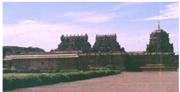
Fig. 3.85. Tanjur. Rajarajeshvara temple. Side view. 1003-1014. Granite.
