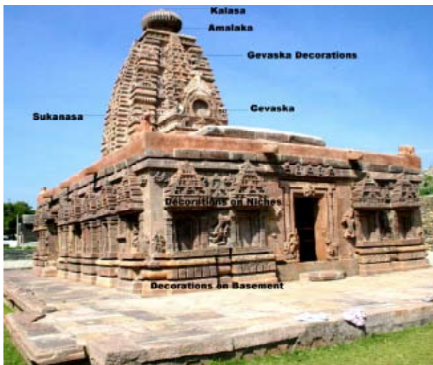
Fig. B. Shape and decoration of North Indian temple tower and temple walls. Visva-Brahma Temple. Alampur. 8 th Century. Sandstone.
