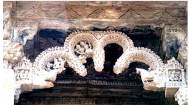
Fig. 3.73. Khajuraho. Kandariya temple. Arch on entrance porch. 1002-35. Sandstone.
