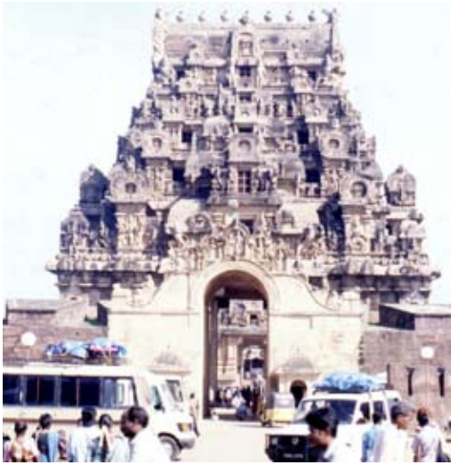
Fig. 3.86. Tanjur. Rajarajeshvara Temple. Outer gateway. 1003-1014. Granite & Brick.
