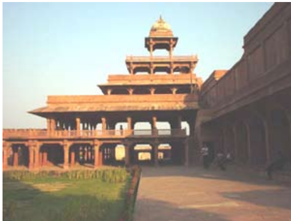
Fig. 5.80. Fatahpursikiri. Panch Mahal. 1572-1575. Sandstone.
