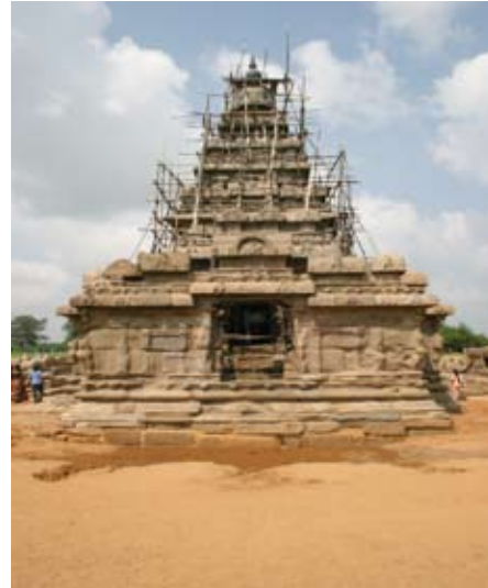
Fig. 2.236. Mamalapurum. Shore temple. Siva shrine facing sea. 8 th Century. Granite.
