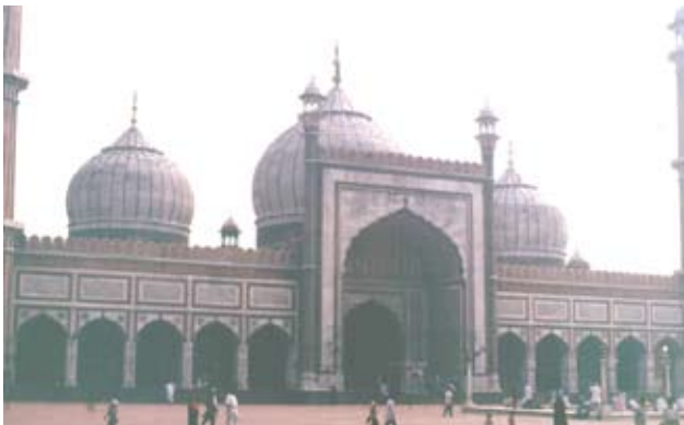
Fig. 5.26. Delhi. Jami Masjid. Façade. 1650-1656. Sandstone.
