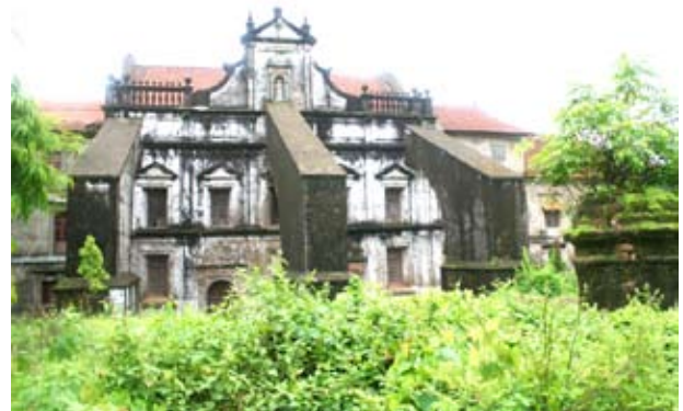
Fig. 5.129. Old Goa. Church and Convent of Saint Monica. Façade. 1606-1627. Laterite and mortar.
