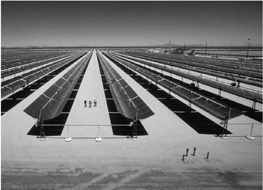
Figure 87: Kramer Junction's SEGS system in California.
