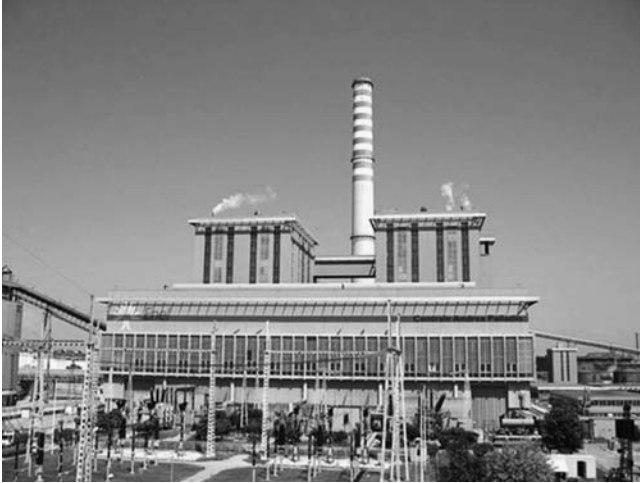
Figure 108: ENEL Priolo Gargallo thermoelectric central scenerly.
