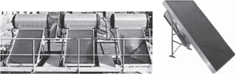
Figure 42: Natural circulation collectors with storage tanks above and behind the panel.
