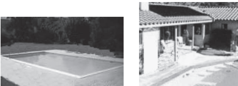
Figure 18: Unglazed panels used to warm up a swimming pool.
