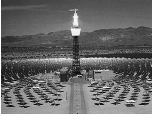
Figure 92: Impianto Solar Two .
