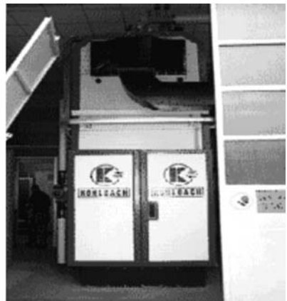
Figure 27: Little-medium power chips or pellet powered boiler.
