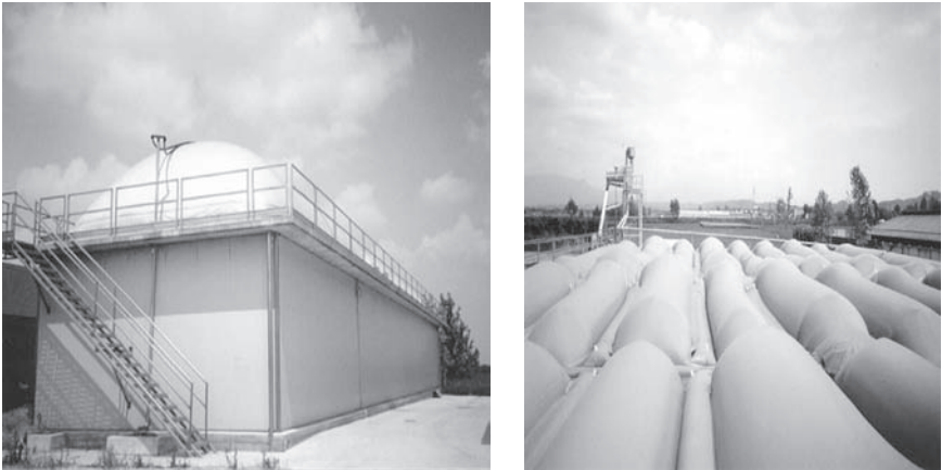
Figure 3: Simplified plant with floating and dome covers.
