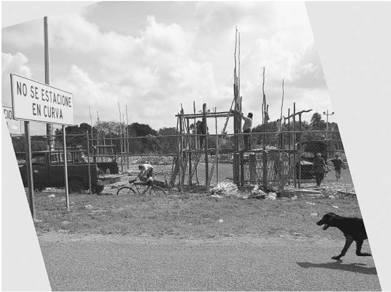
Dismantling bullfight arena
