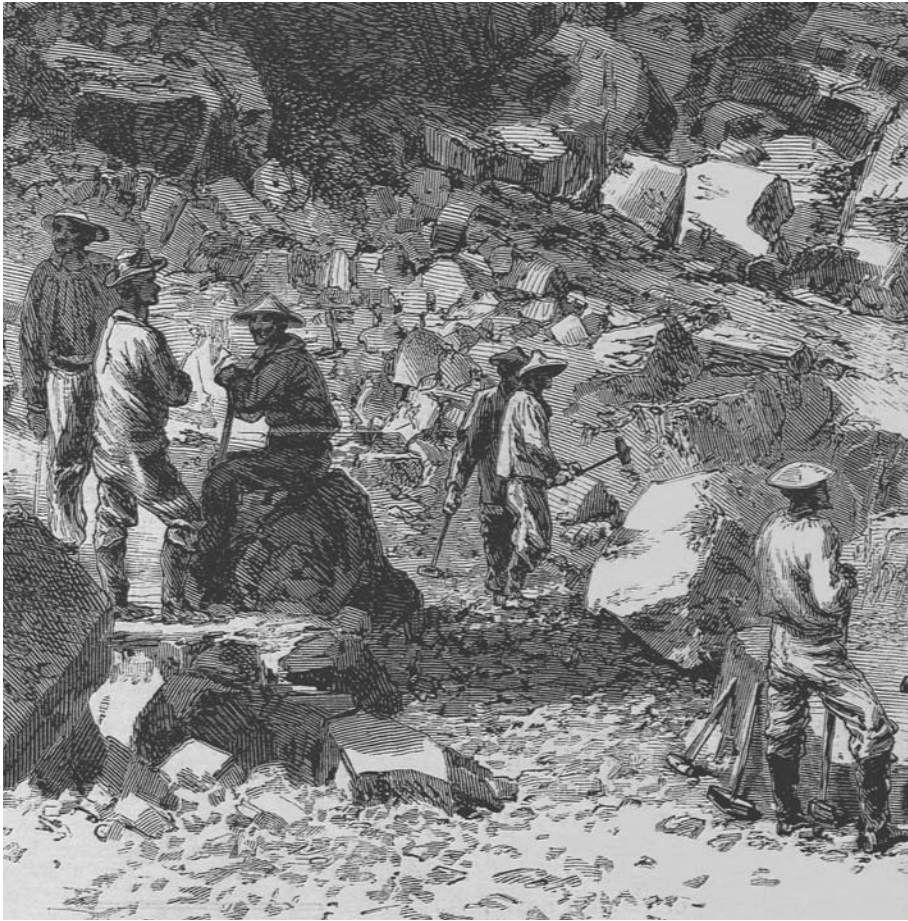
Chinese laborers move rocks to make a path through the mountains for the Central Pacific railroad line.
