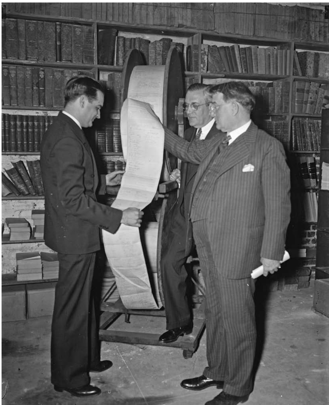
After being received by Congress, Colonel Pope's "Monster Petition" for good roads sat in the basement of the Capitol for over forty years until 1937 when it was moved to the National Archives. Here (viewers L-R) Frank McCallister of the National Archives, Edwin Halsey, the Secretary of State, and Sen. Kenneth McKeller look it over before the move. It has been exhibited several times since, most recently in 2008-09 (photograph by Harris & Ewing for the National Archives. Library of Congress Call No. LC-H22 D 1389 [P&P]).
