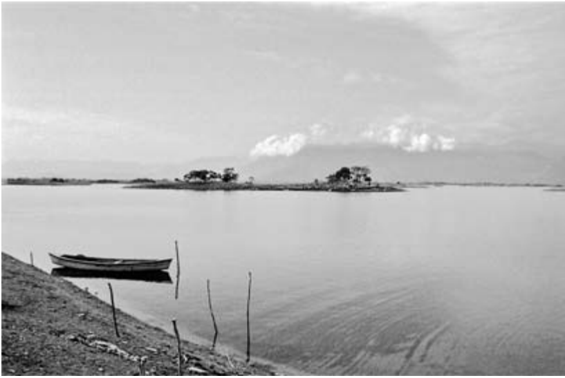
FIGURE 1.3. The reservoir of the Presa Miguel Alemán in the Mazateca Baja, with the Sierra Mazateca in the background.
