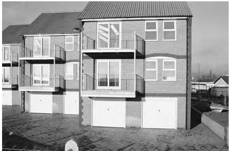
5.6 Boathouse Development Ltd, Jaywick Sands, Essex. Phelen Construction Ltd constructed eighteen seafront apartments in 2003 in Jaywick Sands, a small coastal settlement near Clacton-on-Sea in Essex. The site is located in a place that has suffered from several floods due to high tides and/or storm waters breaching the sea defences. The area remains at risk from flooding. The development incorporates design features that are not dissimilar to those found in most town houses. The two-bedroom apartments are positioned on the first and second floors of the development, and they have a ground-floor garage with a connecting door into a utility room and common stairway up to the principal entrances. The design of the scheme effectively excludes wheelchair users and other mobility impaired people from ease of access to the dwellings. However, this design was a requirement of The Environment Agency in order to minimize the impact of future flooding on residences.
