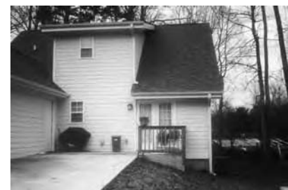
5.14 Providing level access to the back entrance.
