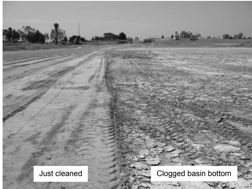
FIGURE 6-3 Clogging layer in recharge basin operated in Orange County, California, adjacent to cleaned portion of recharge basin where the clogging layer was removed. Photo courtesy of Adam Hutchinson, Orange County Water District.
