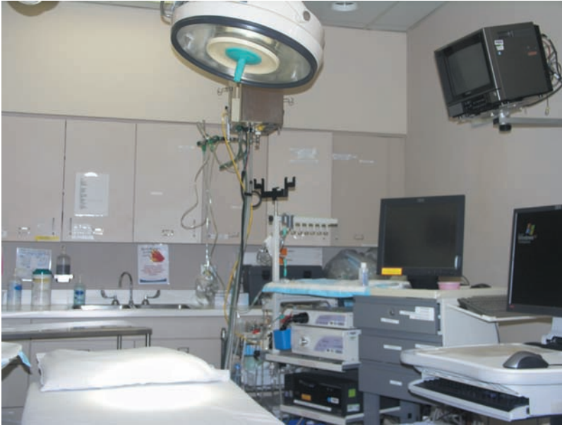
FIGURE 7.7. In some facilities, advanced surgical procedures are performed in bronchoscopy rooms, which therefore need adequate overhead surgical lighting and sterile equipment.
