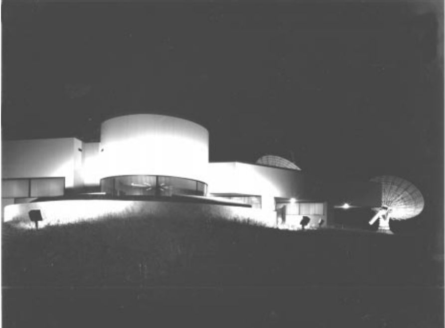
Figure 7.8 The PanAmSat Teleport in Fillmore, CA. (Courtesy of Hughes Electronics Corp.)
