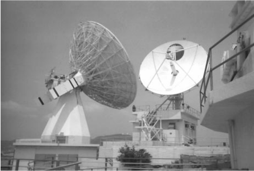
Figure 7.6 INTELSAT earth station antennas in Hong Kong. (Courtesy of Bruce Elbert, Introduction to Satellite Communication, Second Edition , and Hong Kong Telecom.)
