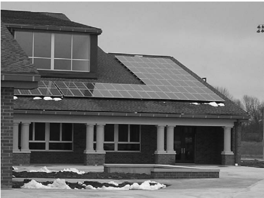
16-7. Solar Collector Array at Twenhofel Middle School, KY
