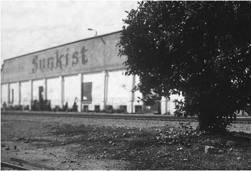
Figure 31. Local residents and former growers, pickers and packers of oranges turned out to witness and lament the demolition of this packing house in Placentia, shown here on the eve of its destruction on February 7, 1997. Many Californians see the loss of agricultural lands to urban and suburban development as a sign that Eden has been lost, but the garden that is gone was itself an expression of an earlier phase of development. (Photograph by the author.)
