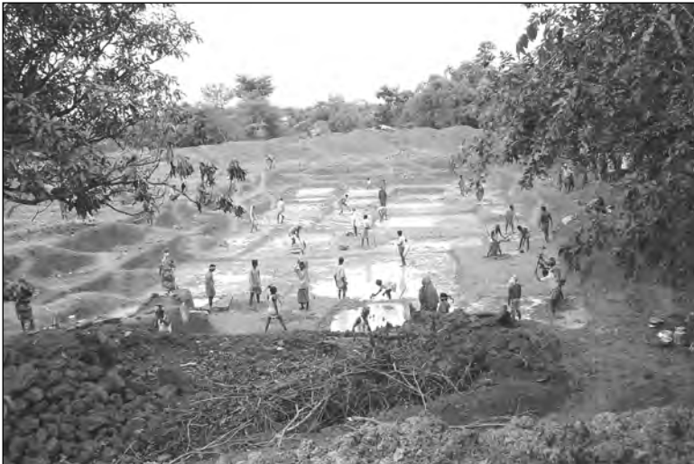
Plate 12.1 A tank being excavated in Tarkilata
