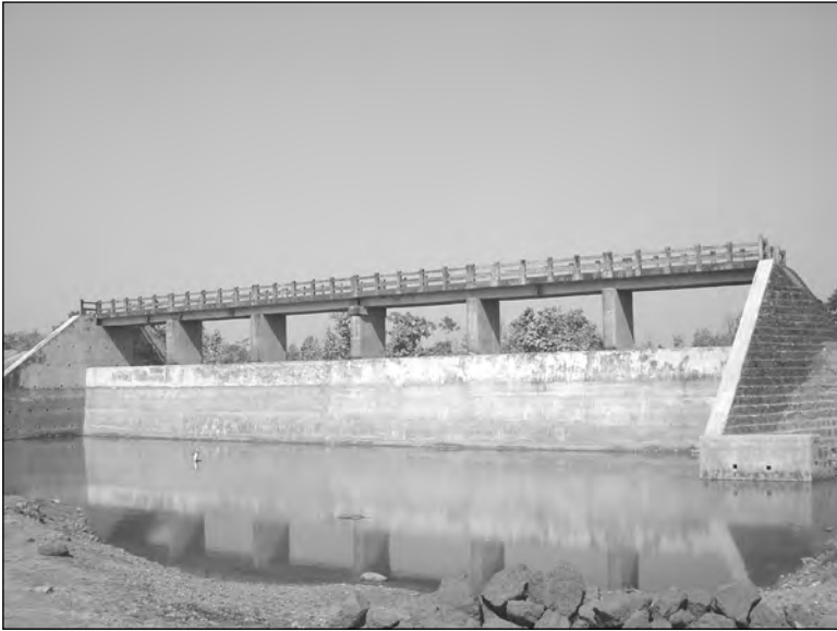
Plate 32.1 The incomplete dam
