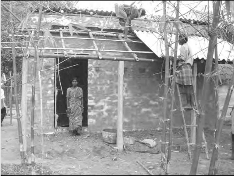
Plate 27.1 Pramila Sabar's house under construction
