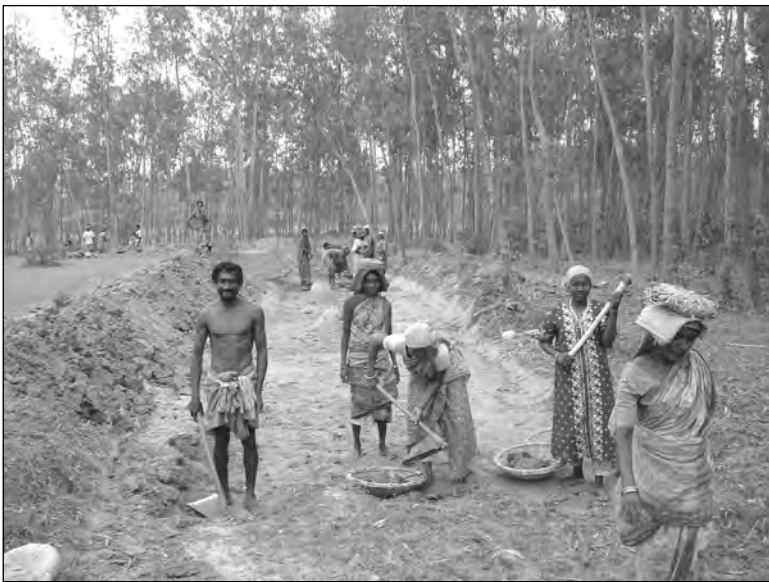
Plate 29.2 A field channel for the overflow
