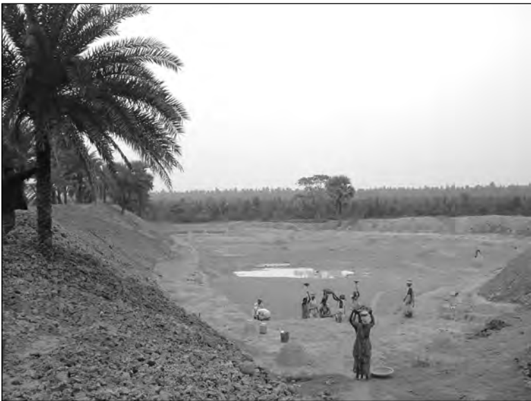
Plate 29.1 Kumar bundh — work in progress
