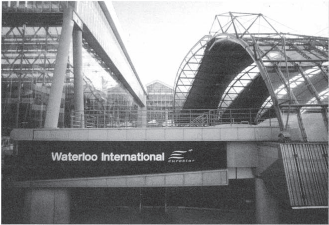
PLATE 1.5 Waterloo International train terminal, London (Jeremy Horner/The Hutchison Library)
