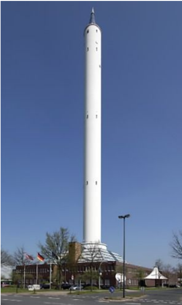
Figure 4 The 140-metre drop tower in Bremen, Germany.
