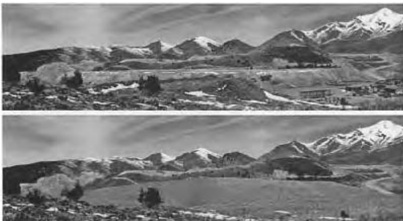
8.2 Barrick-Mercur Mine panoramic view: (top) existing condition; (below) visual simulation after regrading and revegetation
