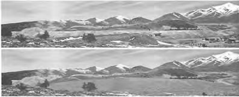
8.2 Barrick-Mercur Mine panoramic view: (top) existing condition; (below) visual simulation after regrading and revegetation (images reproduced in the colour plate section)
