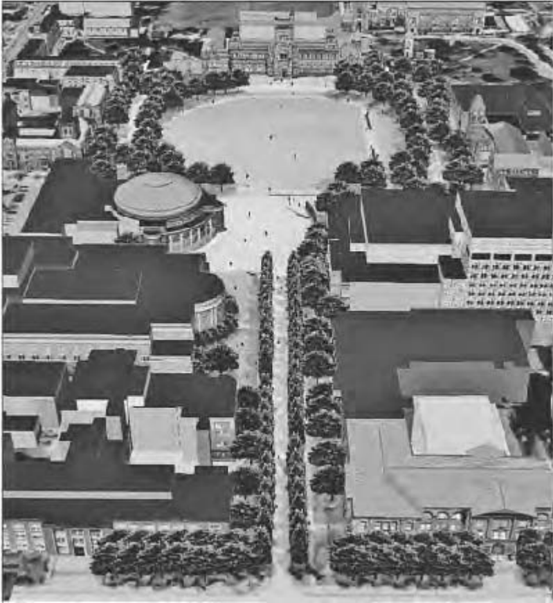
9.10 An aerial overview of the University of Toronto Landscape Open Space Master Plan Concept designed by Urban Strategies Inc. Models such as this one become useful if one can freely look about and move around at eye level, comparing visual concerns with systematic economic and planning parameters that affect feasibility and profit
