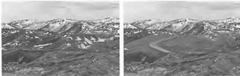
8.3 Barrick-Mercur Mine north side: (left) existing condition; (right) visual simulation after proposed drainage and adjusted road alignment. Pockets of snow were simulated to show the shape and form of the proposed drainages
