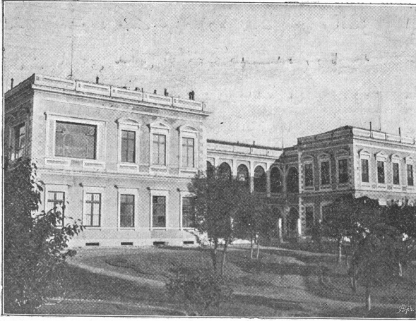
Figure 2 Zeynep-Kamil Hospital in Üsküdar Istanbul
