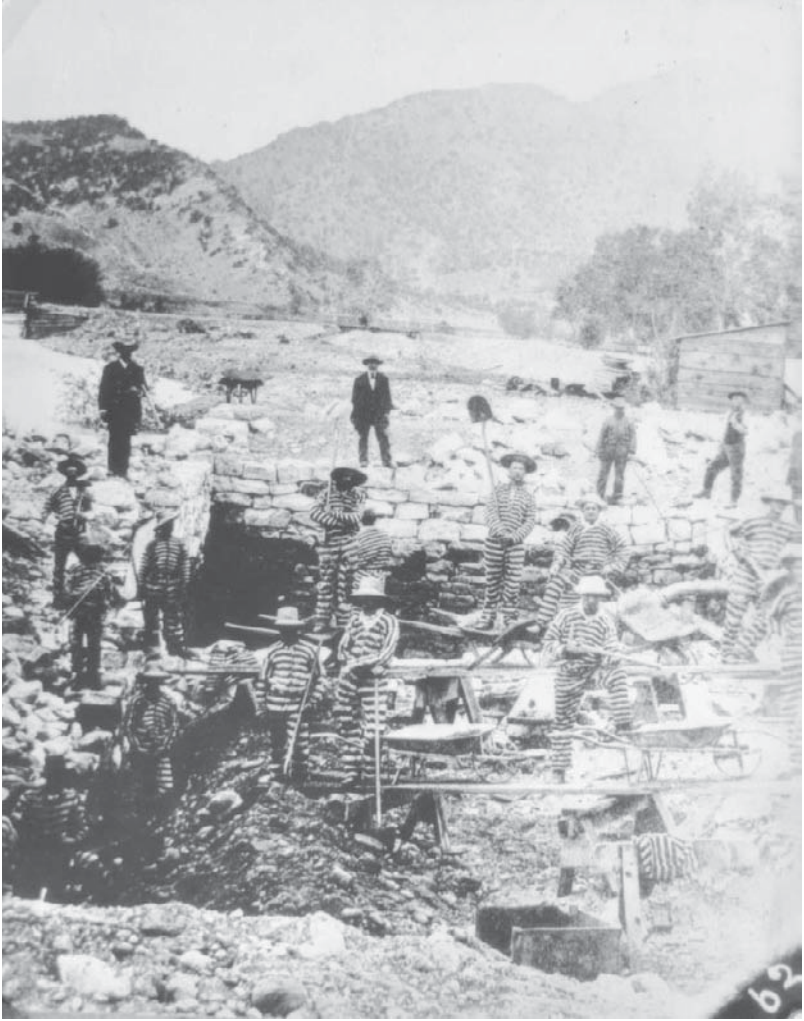
State prisoners excavating the site of a water works in Canon City, Colorado. Convict leasing was most notorious in the South, where disproportionately African American prisoners suffered from overwork and abuse. Photo courtesy of the Western History/Genealogy Department, Denver Public Library.
