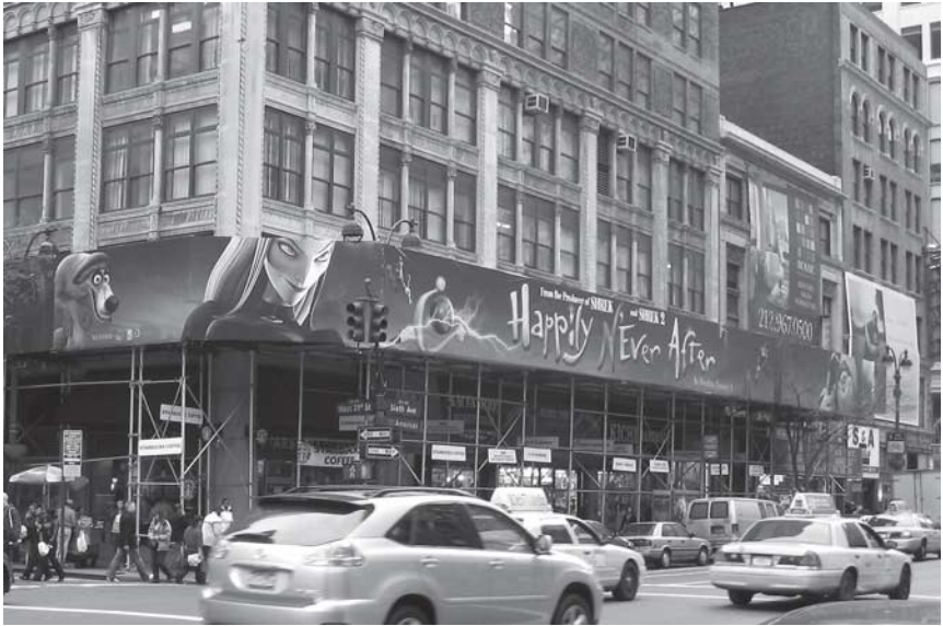
Fig. 10.1. A shed ad, which is also called a construction wrap, is plastered on the side of protective scaffolding for Lionsgate's 2007 animated children's film Happily N'Ever After in New York City. Outdoor ads are ideal for reaching a concentration of urban dwellers. Photo by Robert Marich.
