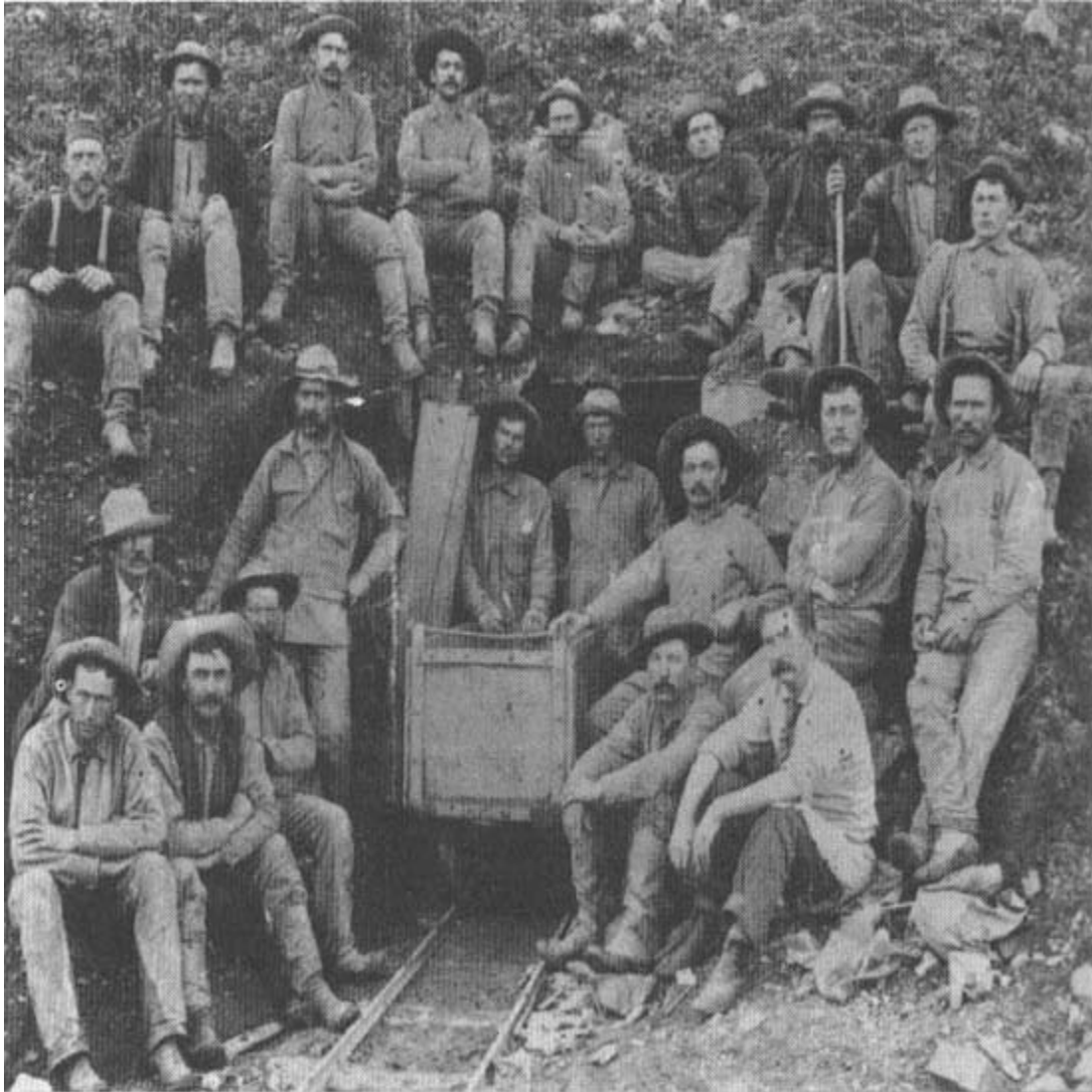
The transition to underground mining: miners in Colorado. Courtesy Colorado Historical Society
