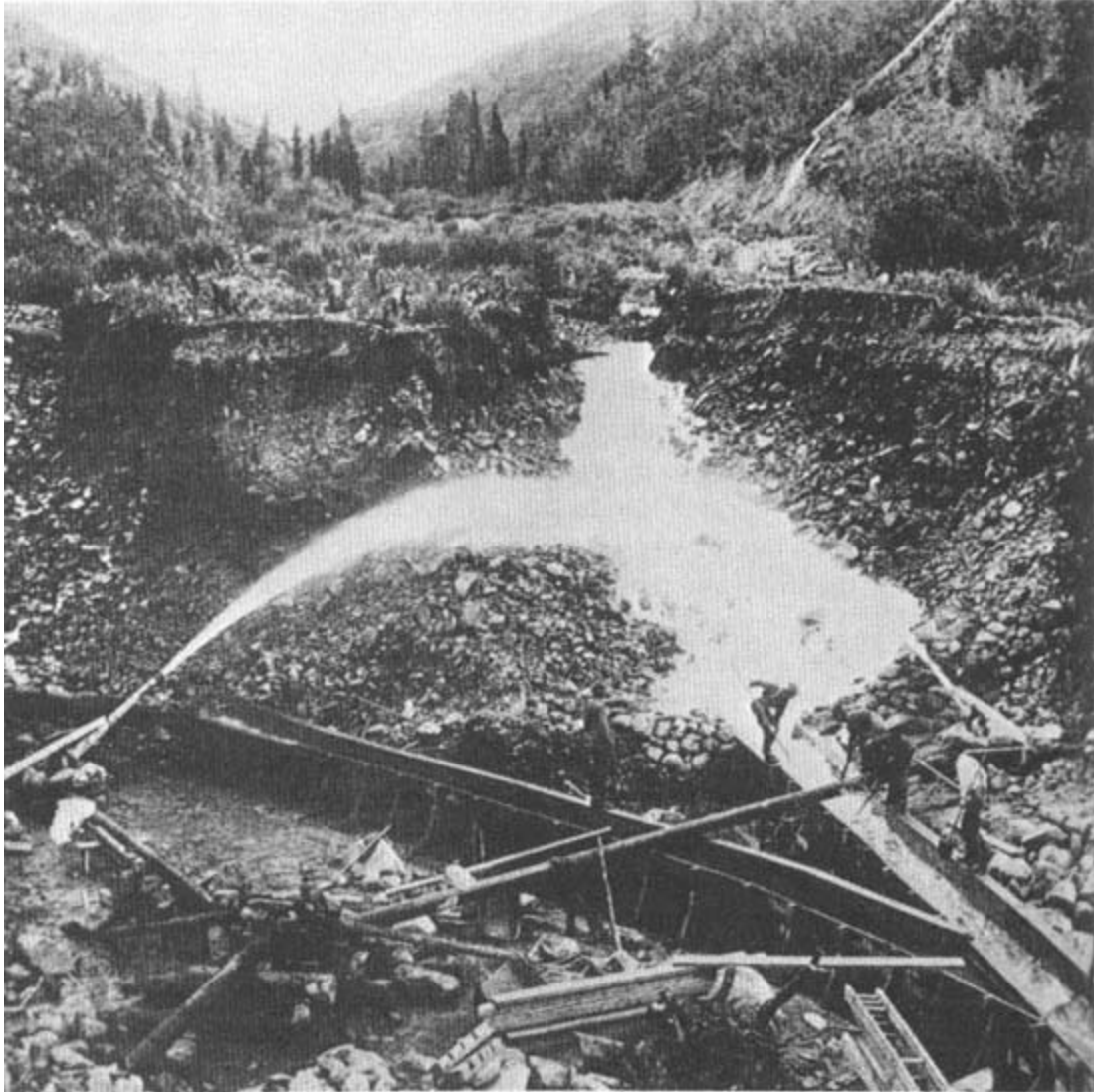
Hydraulic miners transforming a mountain landscape. Courtesy Denver Public Library, Western History Department
