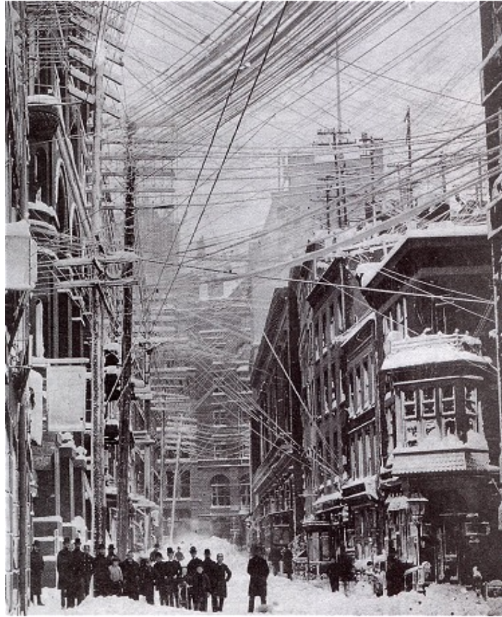
An 1888 blizzard in New York, highlighting a number of telephone, telegraph, and electrical wires. https://commons.wikimedia.org
