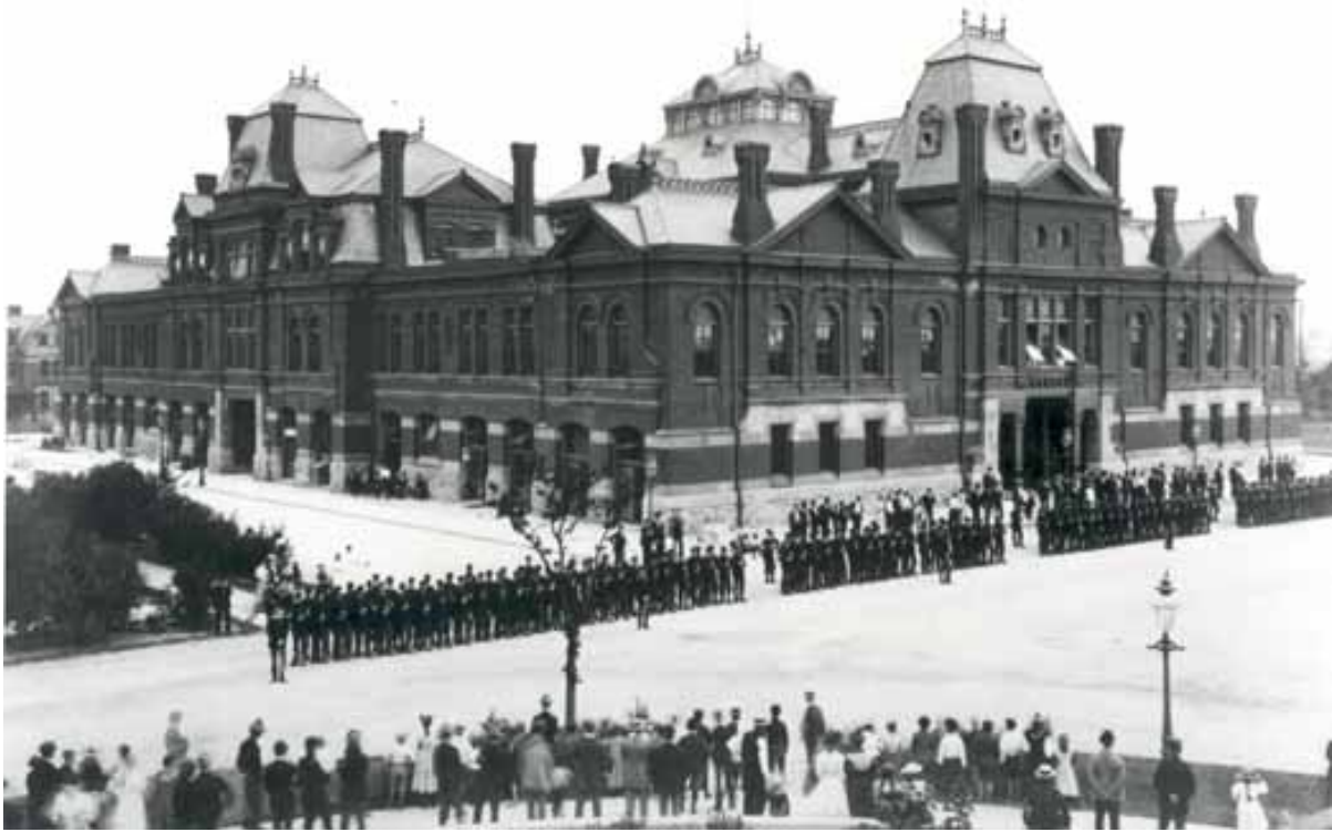
National Guard protecting a factory during the Pullman strike. Source: https://commons.wikimedia.org
