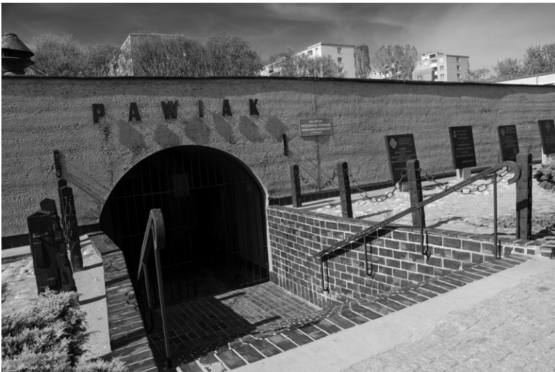
Figure 5.1. Pawiak Prison, a prison built in 1835 in Warsaw, Poland, and used by the Gestapo during World War II. Since 1990, it has been the Museum of Prison Pawiak. Photo by iStock/piotrbb.
