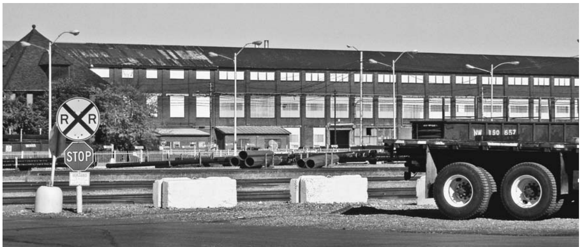
The steel plant where George Wofford, Chloe Wofford's (Toni Morrison's) father worked during her childhood ( Photograph by Carmen R. Gillespie )
