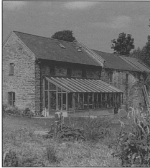
Plate 12. Old Mill, Crossgar (South & East elevations)
