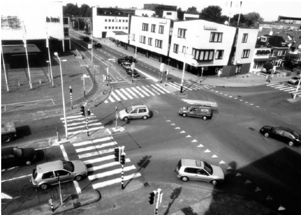
The Laweiplein intersection, before © Knowledge Center Shared Space
