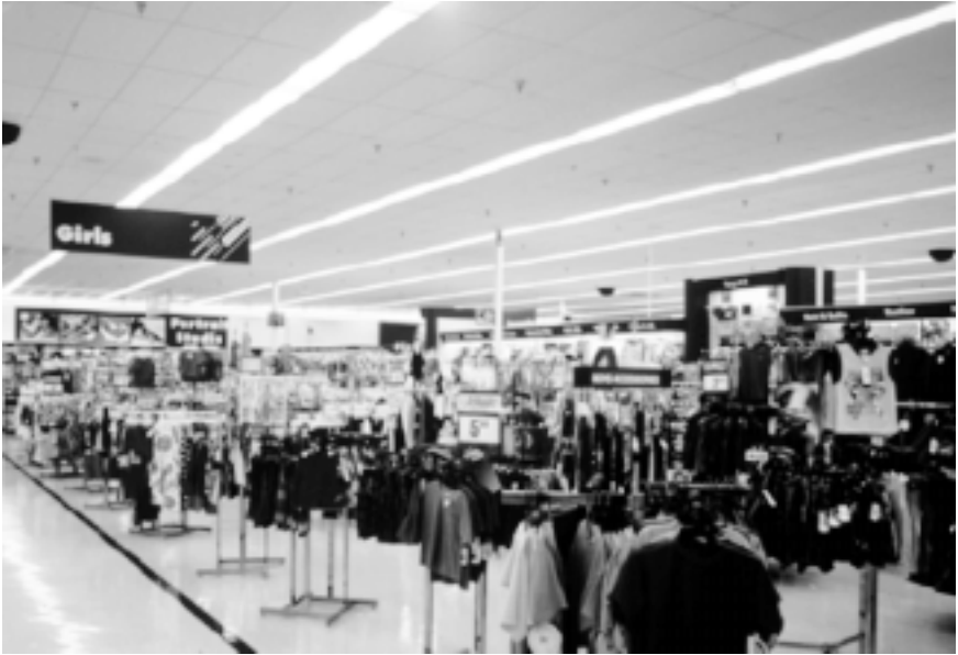
Figure 15-1. High-activity stores maintain relatively high light levels with few (if any) feature displays. Courtesy: Lithonia Lighting.
