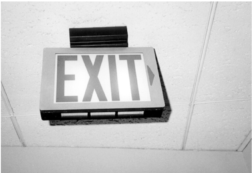
Figure 9-2. A panel exit sign is easily identified by its luminous panel; both the letters and the background are illuminated. Only white light sources should be used in these types of exit signs.
