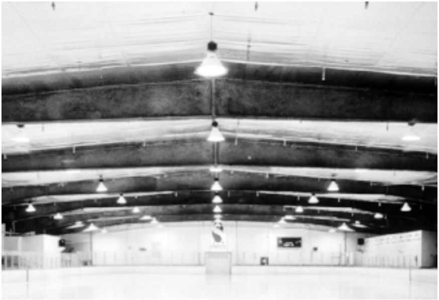
Figure 8-5. High-bay compact fluorescent luminaires are effective in indoor sports arenas, particularly where the ceiling is relatively low compared to the length and width of the room. These luminaires provide good vertical illumination, and with the use of high-frequency electronic ballasts, these light sources do not cause strobe problems. Courtesy: Sportlite, Inc.
