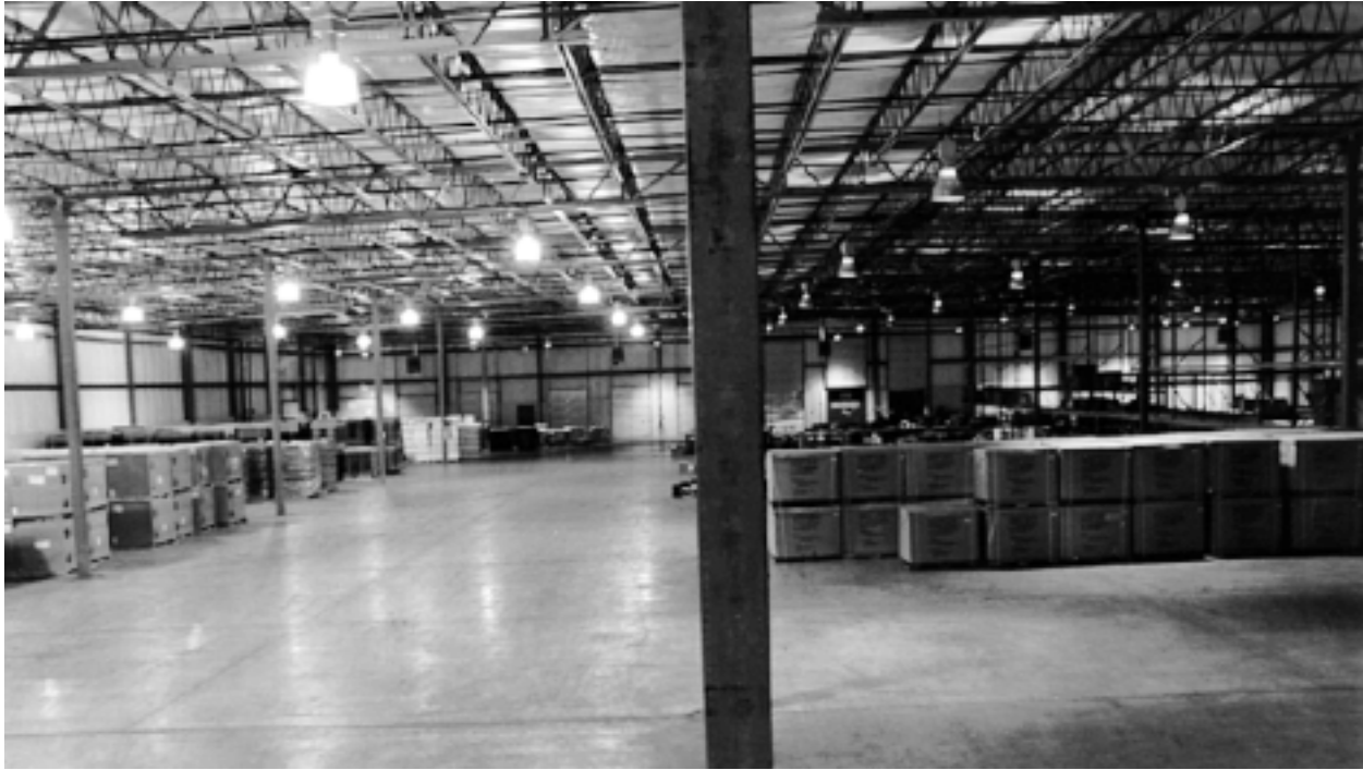
Figure 16-5. Retrofit clear reflectors (shown on left side of photograph) can brighten work surfaces while maximizing luminaire efficiency. Courtesy: Lexalite International.
