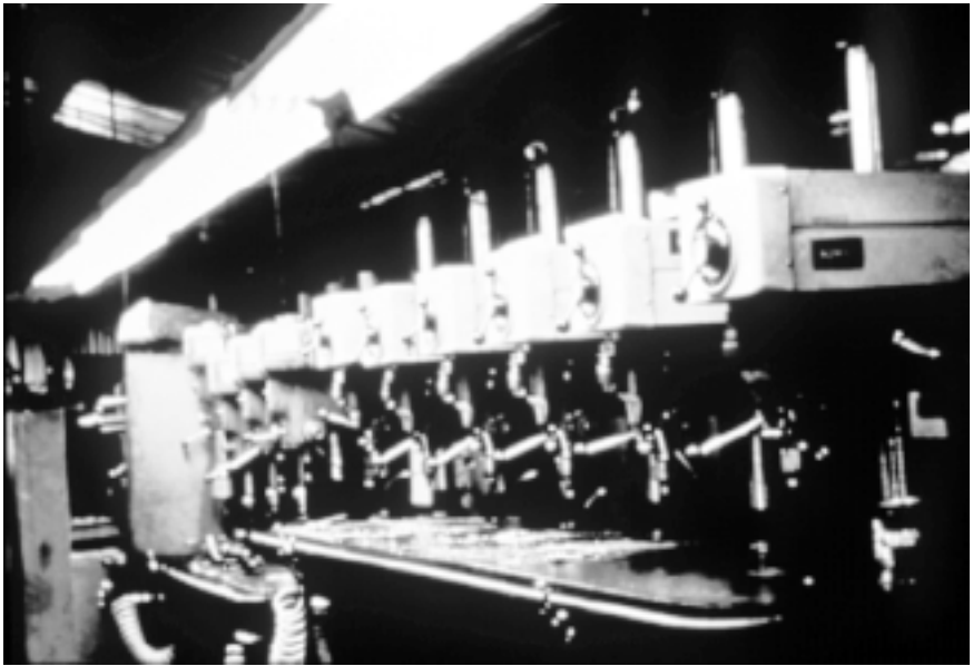
Figure 16-2. Task lighting should be used wherever higher light levels are needed for enhancing safety and productivity. Typical applications include machine operation, inspection and assembly. Courtesy: Illuminating Engineering Society of North America.
