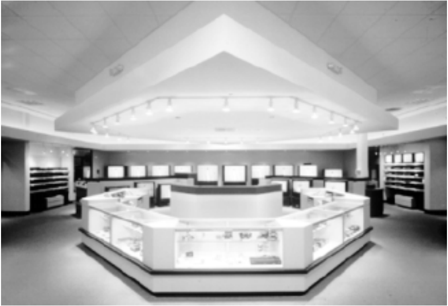
Figure 15-4. Low-activity stores provide maximum glare control and reduced levels of general illumination. Dramatic display lighting is achieved with halogen lamps that provide precise beam control. Courtesy: Philips Lighting Company.
