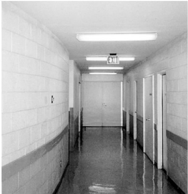
Figure 9-1. In this application, the exit sign marks where there is a change in direction of the exit route.
