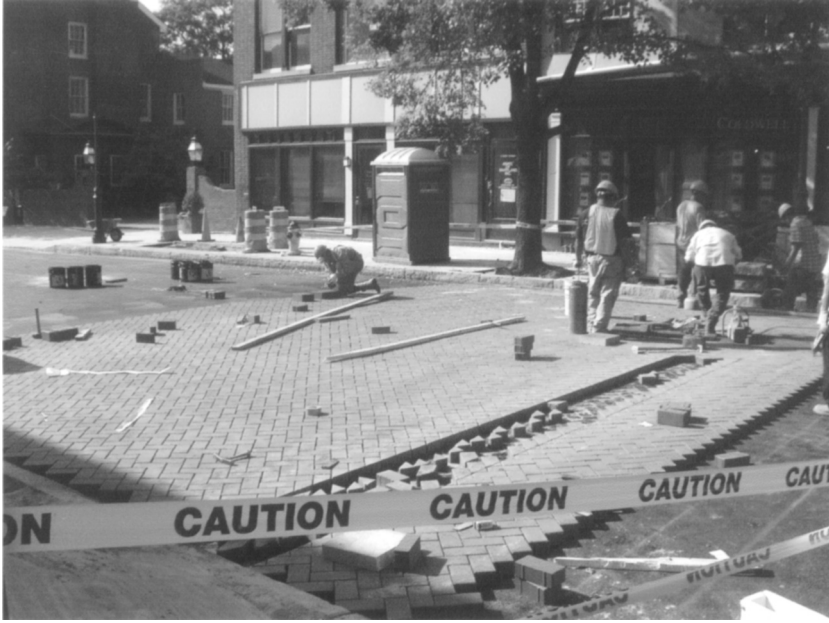
Figure 11.1 Laying brick pavings in the Historic District of Annapolis, Maryland.
