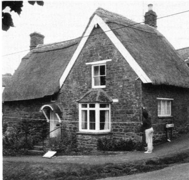
36 (Left) Drawing an elevation of an eighteenth-century cottage at Byfield, Northamptonshire. Because the cottage is built on a slope a levelled line has been put up to measure from.
