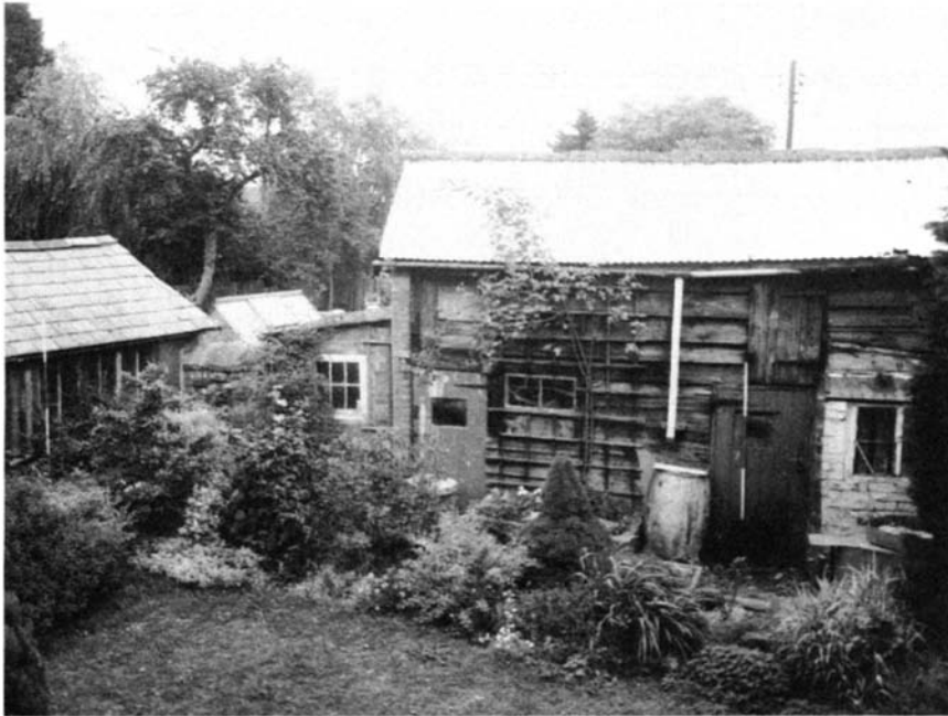
31 Small-scale nineteenth-century 'industrial' buildings, Cropredy, Oxfordshire. On the right a small barn used by the village stone mason, on the left a cobbler's workshop from the 1900s. The path joining the two is made from fragments of gravestones.
