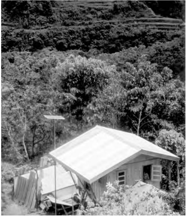
Figure 7.4 Solar home in remote valley in the Philippines
