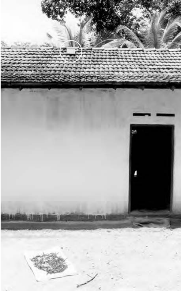
Figure 7.1 Example of a small solar system (10 watts) installed in Sri Lanka
