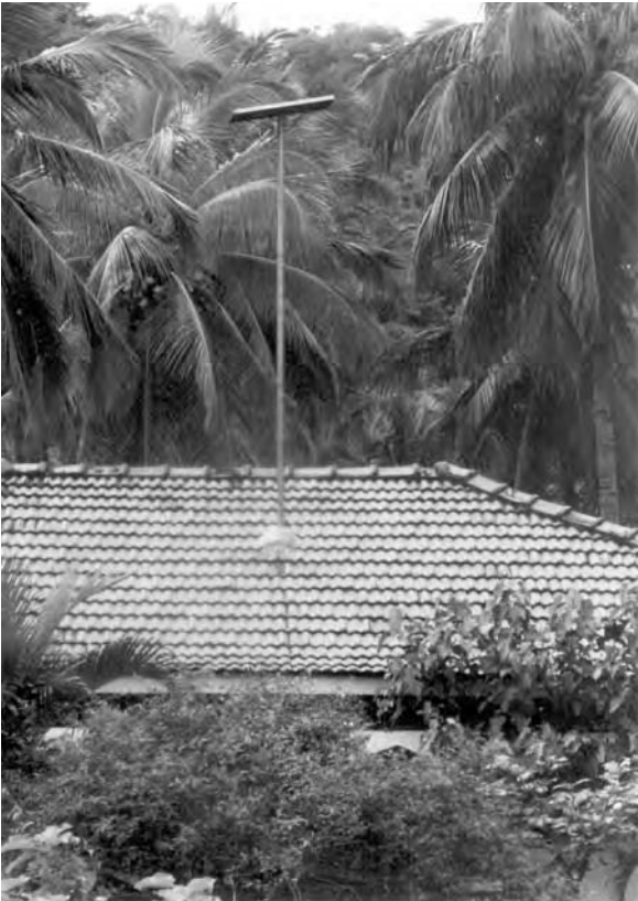
Figure 5.38 Lifting a solar module above shadow caused by trees
