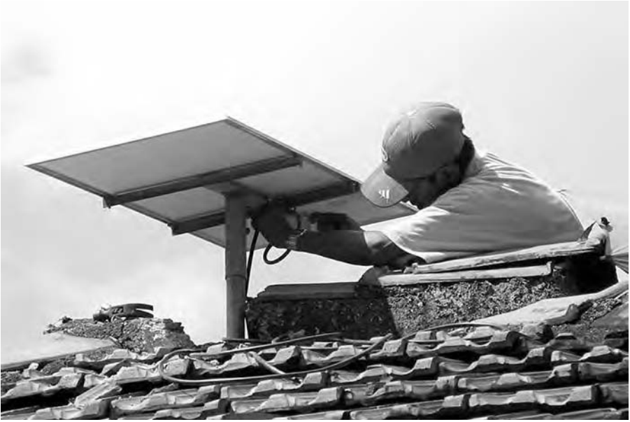
Figure 5.49 Technician installing solar module on rooftop
