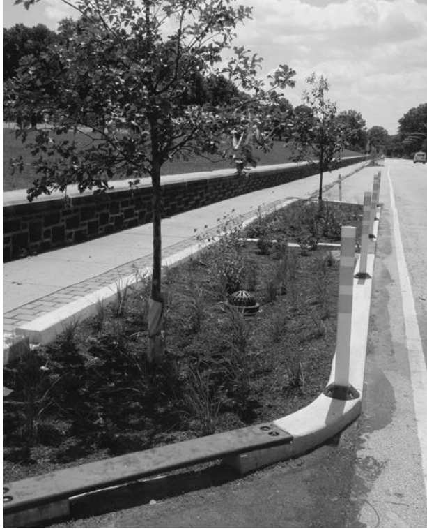
Figure 2.1 Queen Lane stormwater bumpouts.
