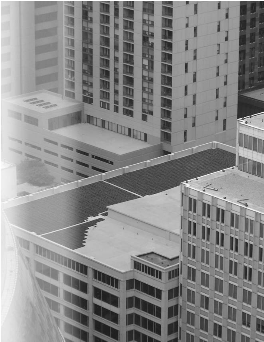
Figure 3.2 Sedum green roof on parking garage, 161 N. Clark, Chicago.
