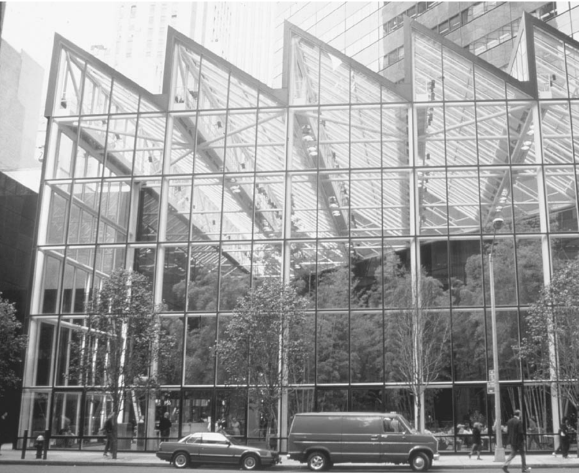
Figure 4.4. Exterior of atrium, 2001.
